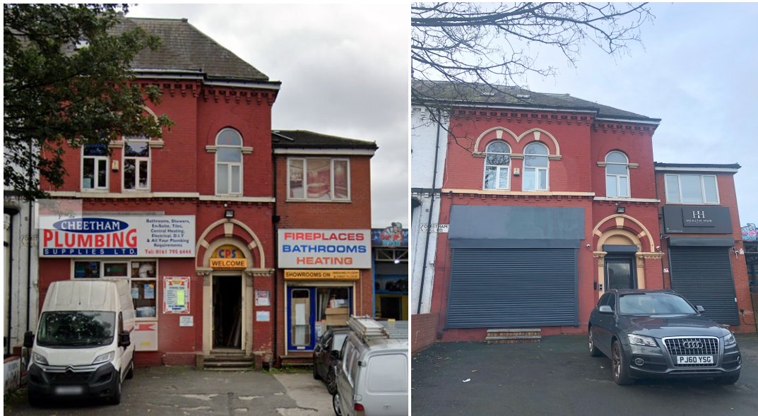
Figure 1, Image of the front elevation – left hand image (August 2021- Google Maps) and right hand image (February 2025- site visit)
