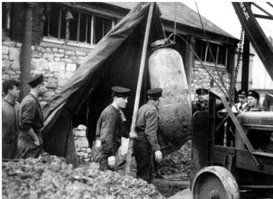
Removal of an UXB
