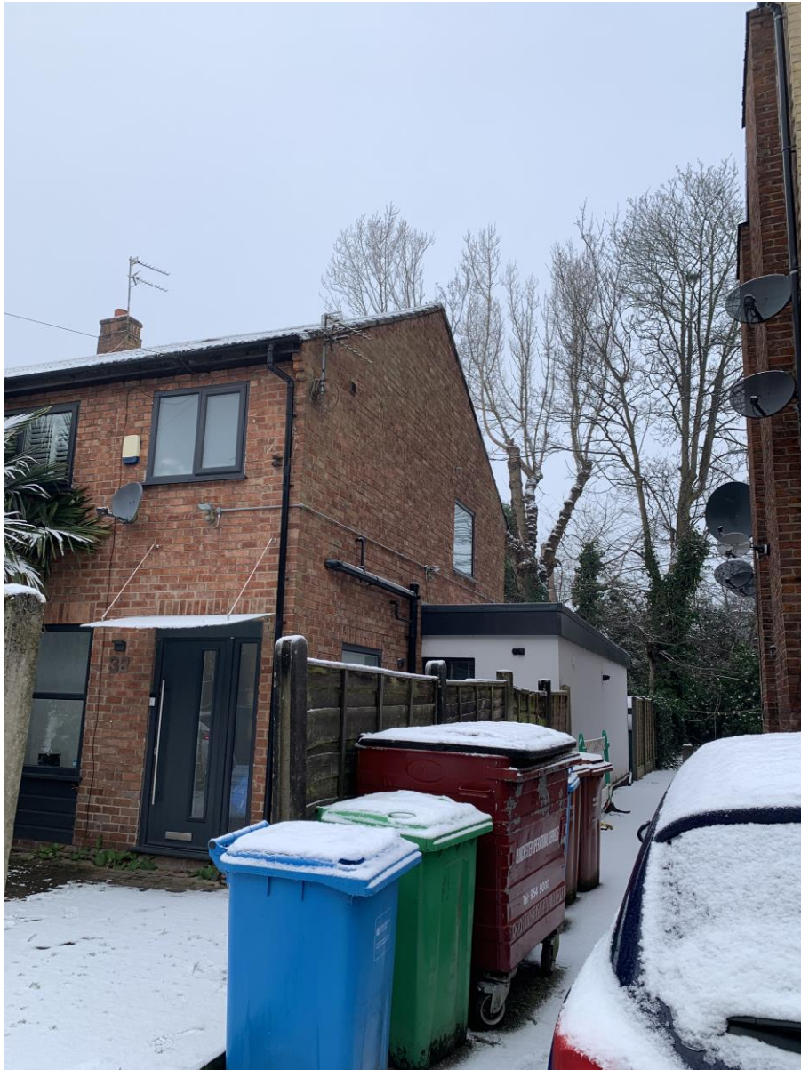
Side view of the 32 Northen Grove
