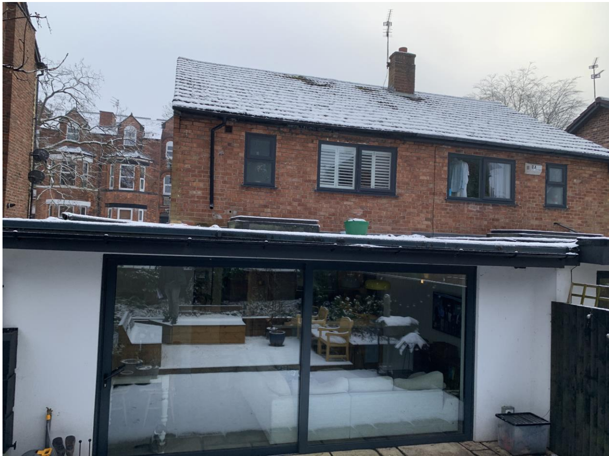
Rear view of the 32 Northen Grove
