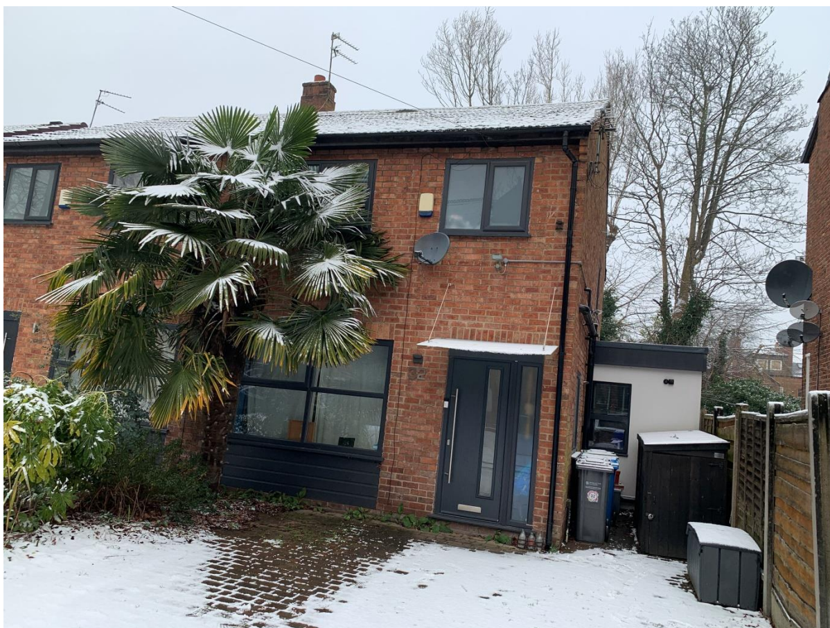
Front view of the 32 Northen Grove.
