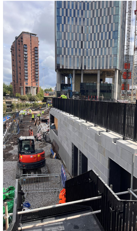
SITE PHOTO - WIDER BALUSTRADE
