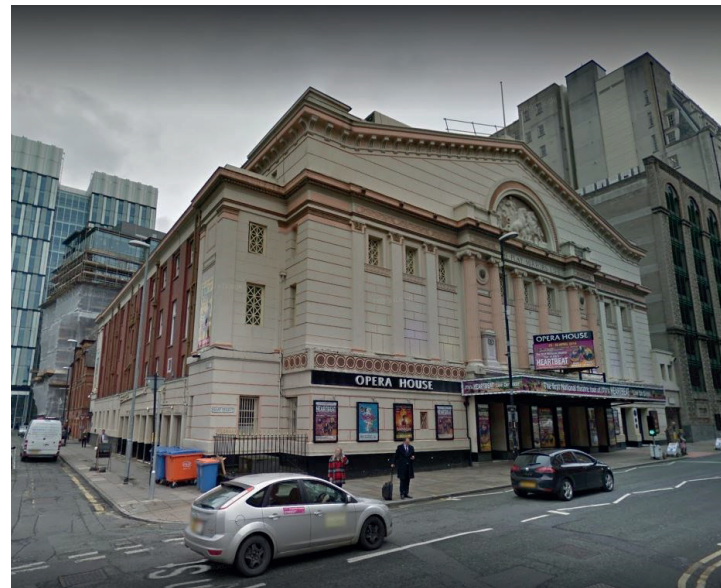
Photograph 3—Current façade (Google Street View)
