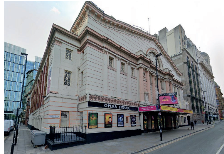
Photograph 6—current façade (google street view)
