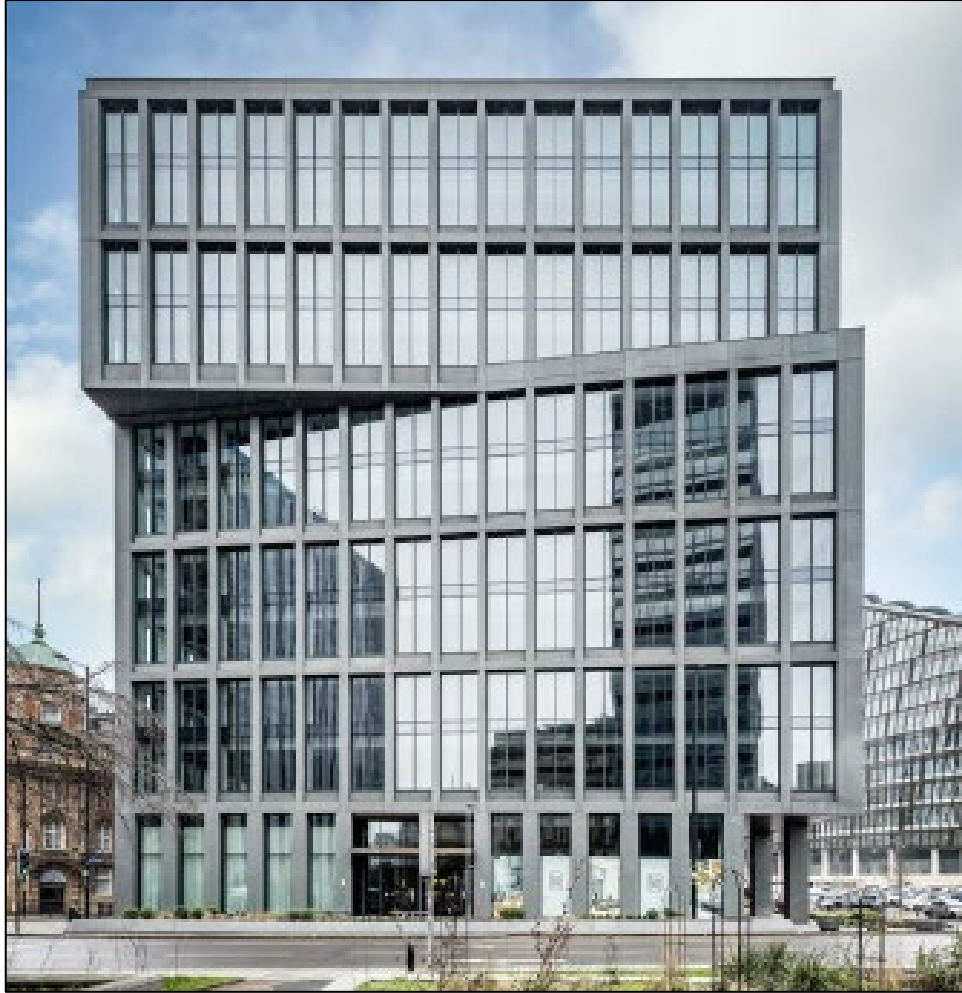
Figure 2: Completed south elevation, showing main entrance
