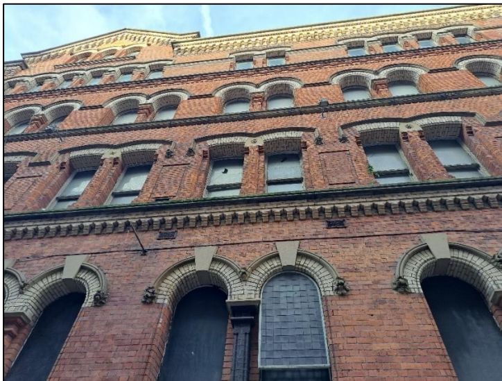
Photograph 1 showing the south-east elevation of the building
