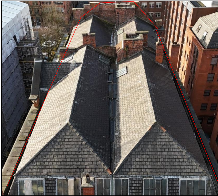
Photograph 2 showing the roof of the building
