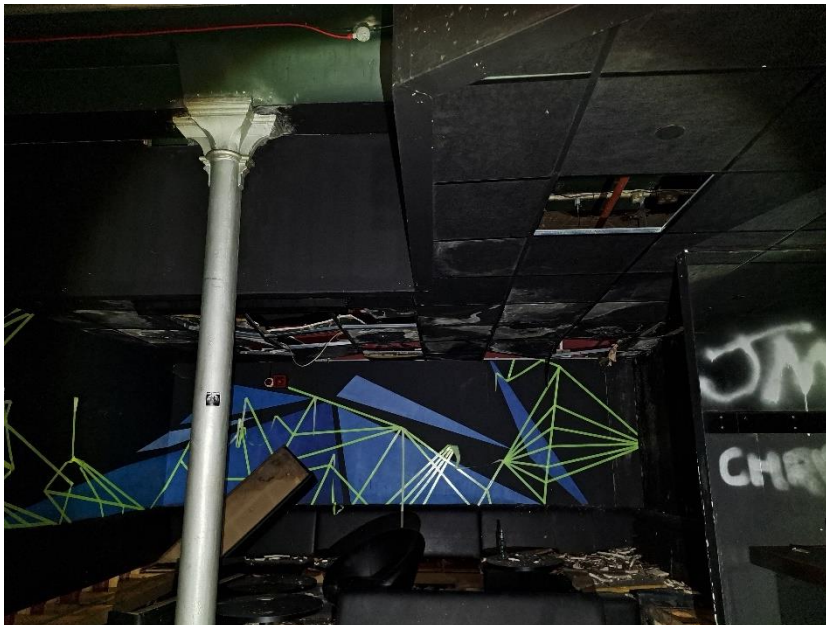
Photograph 7 showing a section of the basement
