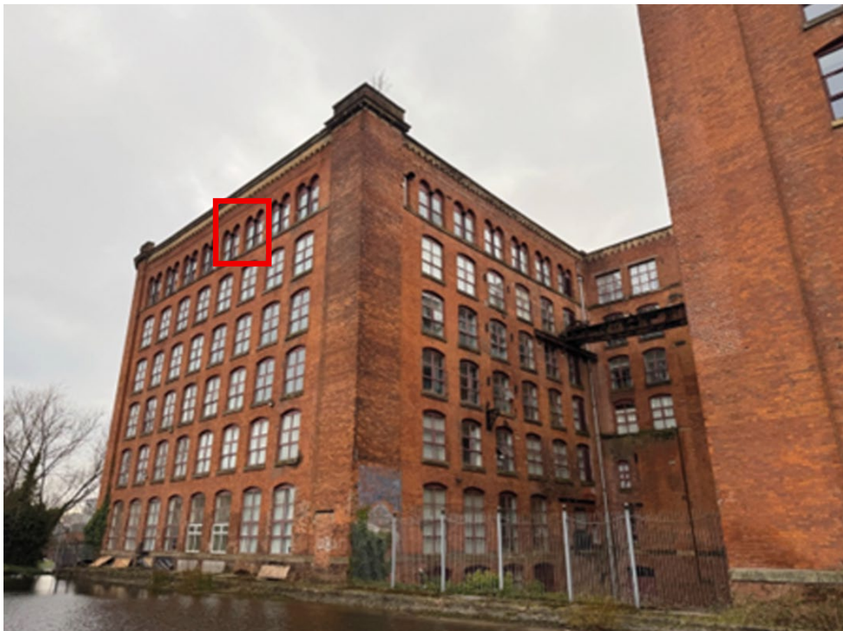
South Elevation showing Fifth Floor timber windows to be replaced along waterfront
