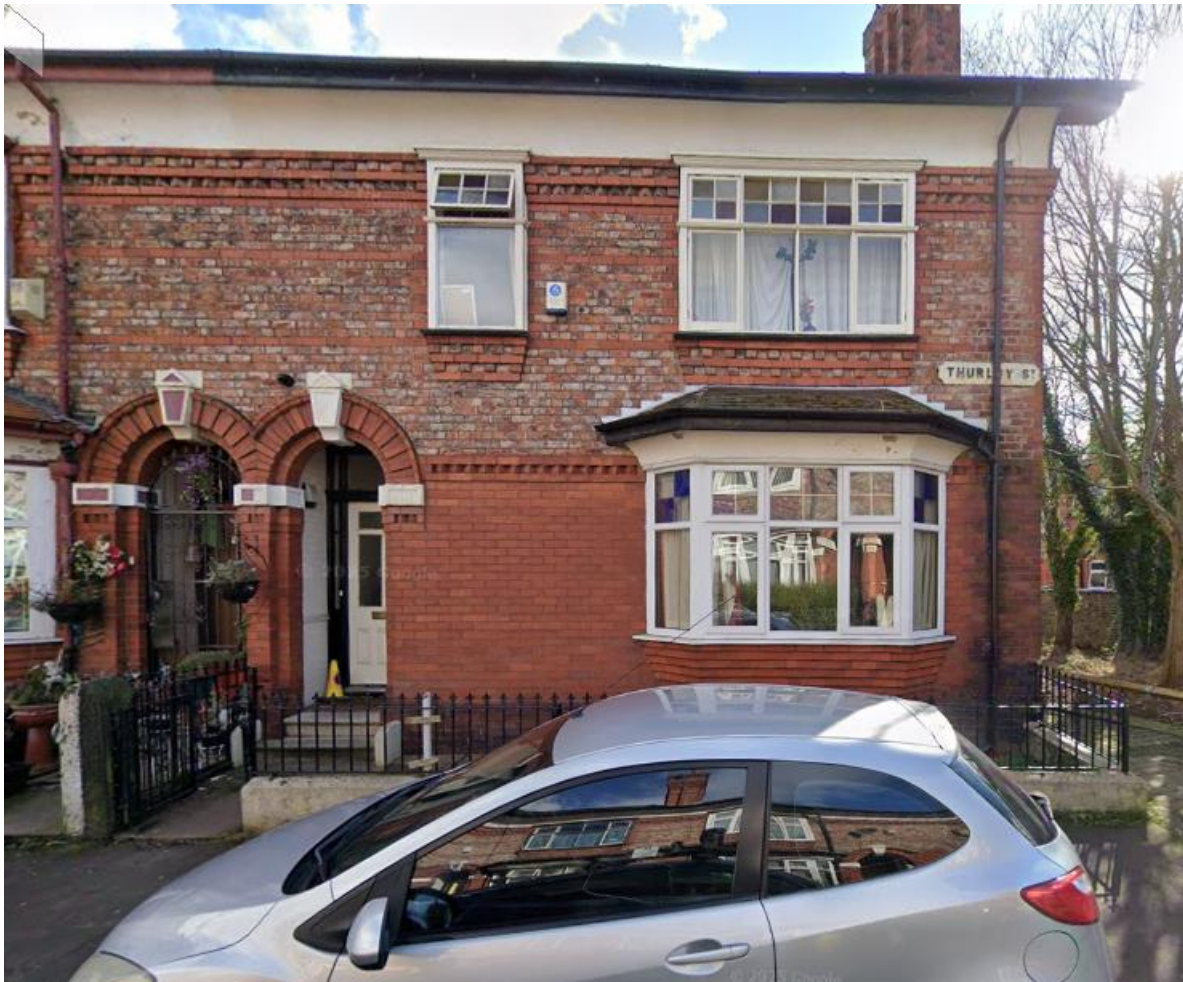
Figure 1. Front Elevation (Google Street View dated March 2025, accessed Sept 2025)
