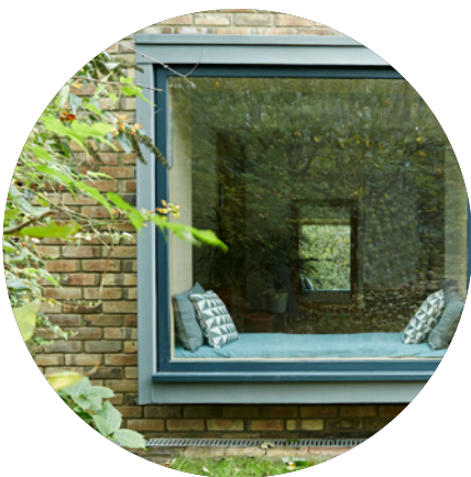
Oriel window with copper coloured surrounds provides a feature to the gable end both internally and externally.
