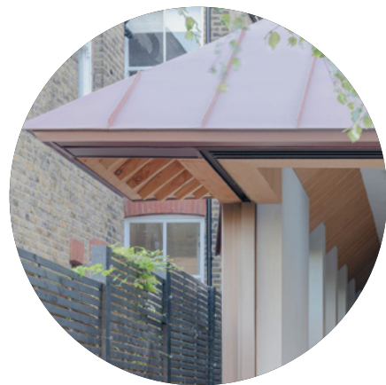
Copper coloured standing seam metal roof is a modern alternative to rosemary tile hipped while maintaining similar colour.
