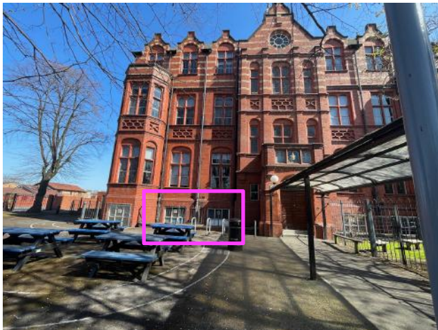
Main Building West elevation, staff toilet windows highlighted.
