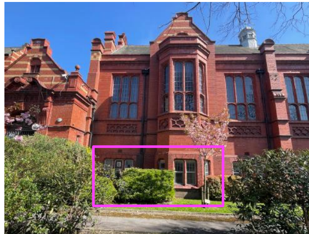
Main Building West elevation, pupil toilet windows highlighted.
