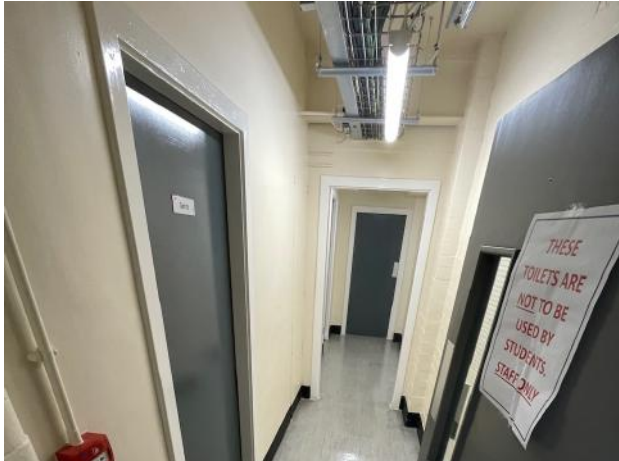
Circulation corridor outside the existing staff toilets
