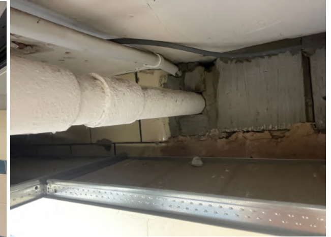
Dividing wall between existing girls and boys toilets showing the original brick wall junction with the modern to be removed.
