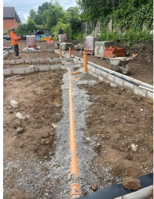
Photo. 02 – General drainage installation
