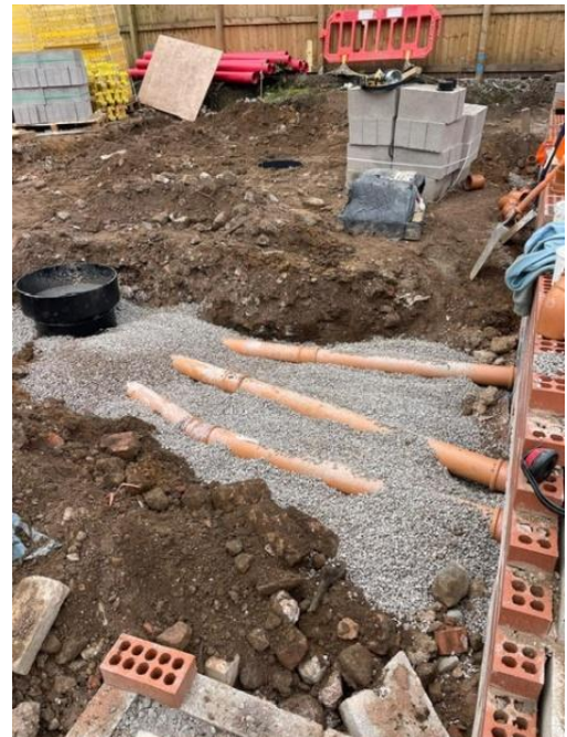
Photo. 04 – General drainage installation
