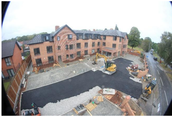
Photo. 05 – Installation of car park
