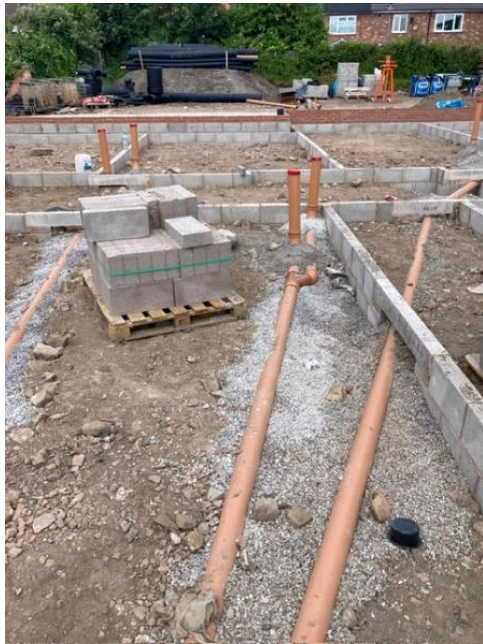
Photo. 01 – General drainage installation
