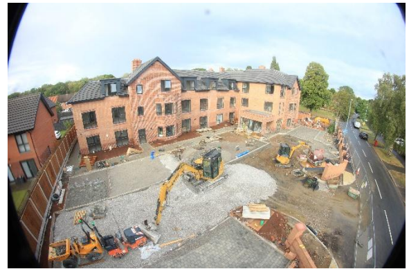
Photo. 06 – Installation of car park
