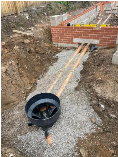
Photo. 03 – General drainage installation
