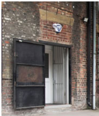
G - Main Entrance The main entrance retains its original lintel. The doorway is infilled with matching brick above a non-original iron door, marking later adaptation.
