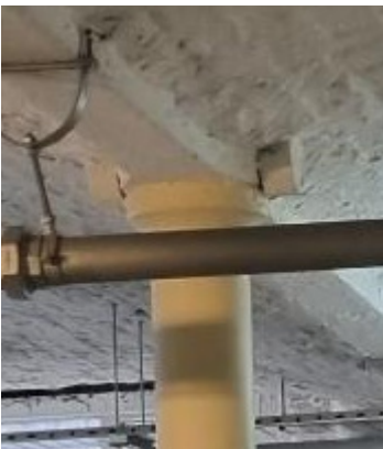
A - Cast-iron beams and columns Cast-iron inverted T-section beams and cylindrical columns support the brick vaults, with exposed tie-rods visible near the beam connections
