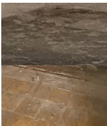
E - Floor Finishes Most of the floors in the mill have been replaced comprising of wooden boards, cement or bitumen. Floor finishes have already been stripped.
