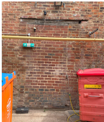
H - Fire Escape (Yard Elevation) No original lintel. Replaced with timber lintel. Previous fire escape door infilled with brick
