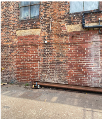
I - Windows (Yard Elevation) Original windows have been lost and infilled. Splayed stone lintels remain as key heritage features.
