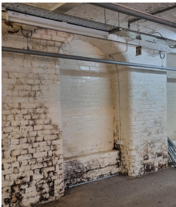
B - Typical step-in window bay This bay demonstrates the 'pier and panel' wall construction, with a typical step-in window opening now infilled with brick.
