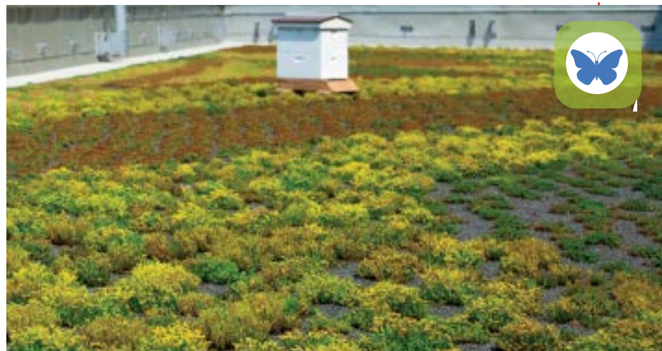
Bands within green roof planting
