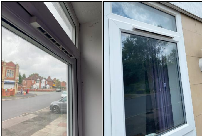
Figure 4.1 - Photographs showing frame-mounted trickle vents, front elevation
