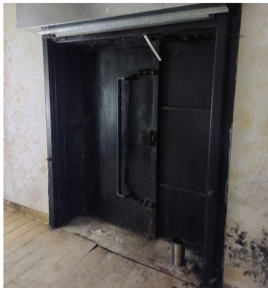
Figure 4.5. Rear exit of the Site at lower level
