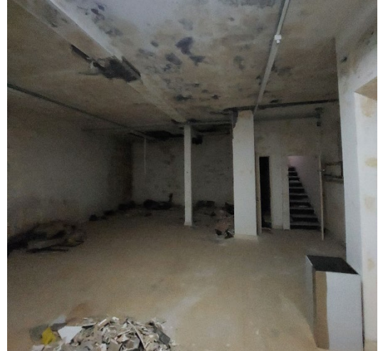
Figure 4.4. Lower floor of the Site
