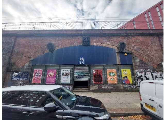
Figure 4.2. Front elevation of Arch 77
