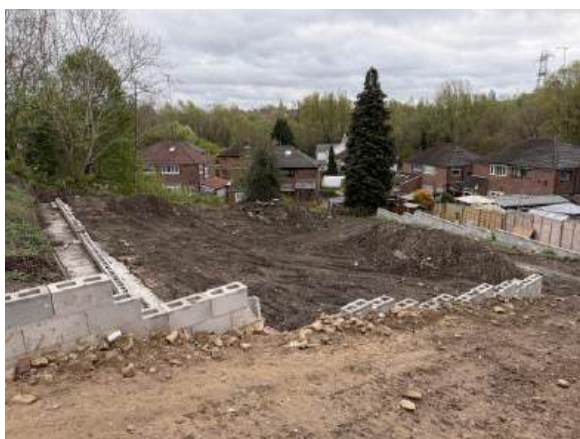
Photograph 1 – Facing south-east of 31 Berry Brow, now cleared for development
