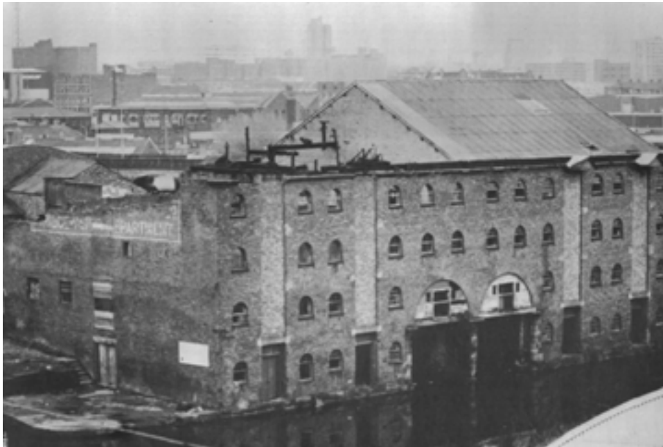
1971 Building condition after fire
