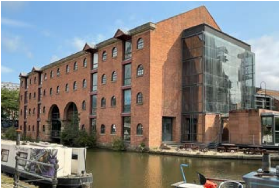
2025 Current condition - west and south elevation
