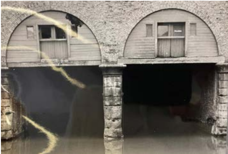
1970 Original shipping hole openings
