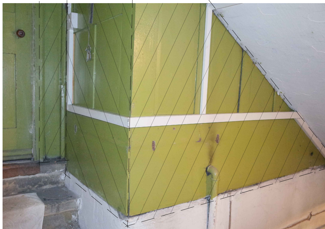
C - Panelling to Basement on south side of stair (nts).
