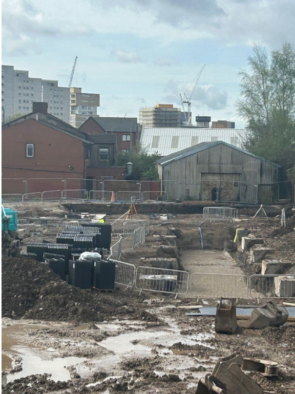
Osbourne Yard 271 Oldham Road, Manchester Attenuation Tank Installation – Photographs 27/10/25
