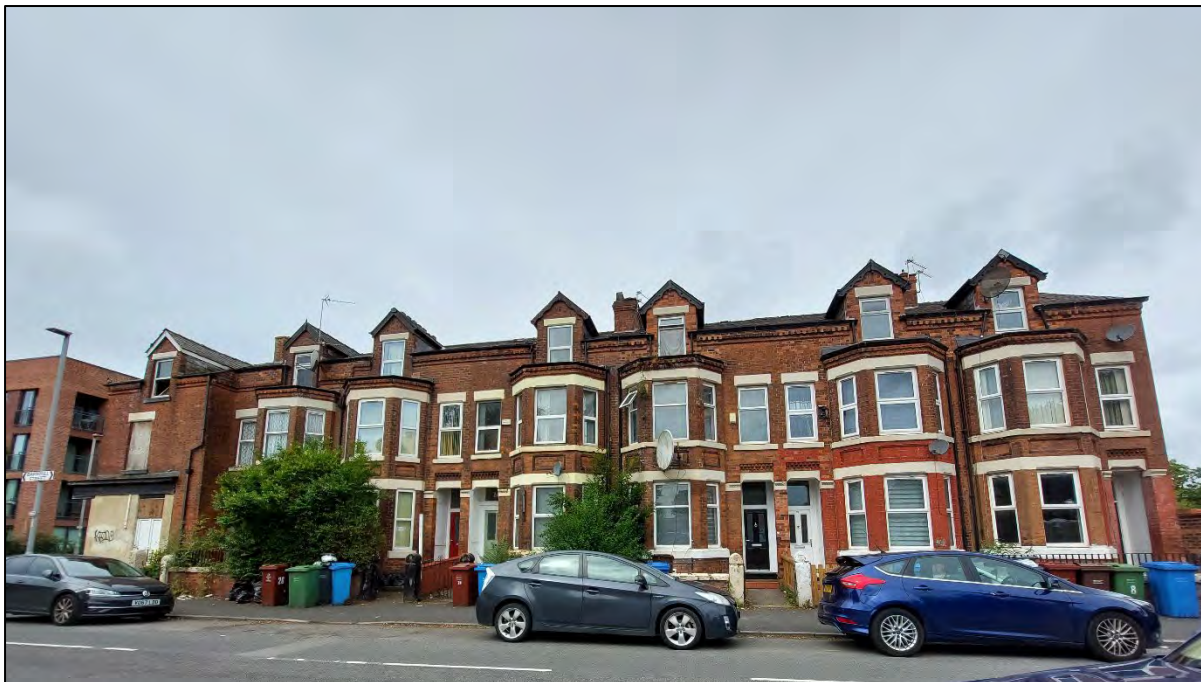
Plate 22 Photograph showing row of terraced houses along Barton Street within Site 1, facing west
