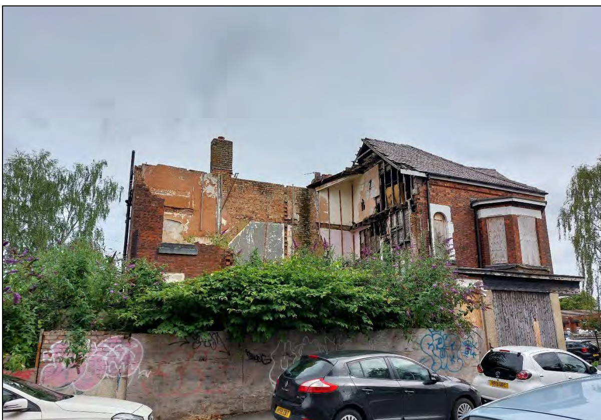
Plate 23 Photograph showing the rear end of the end terraced house at the junction of Barton Street and Raby Street, within Site 1, facing north-east
