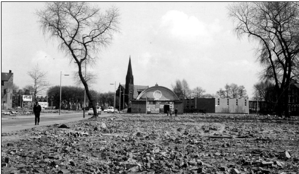
Plate 15 Photograph taken from Barnhill Street showing the Billiards Hall and part of Site 3 to the south, taken in 1972. Courtesy of the Manchester Local Image Collection
