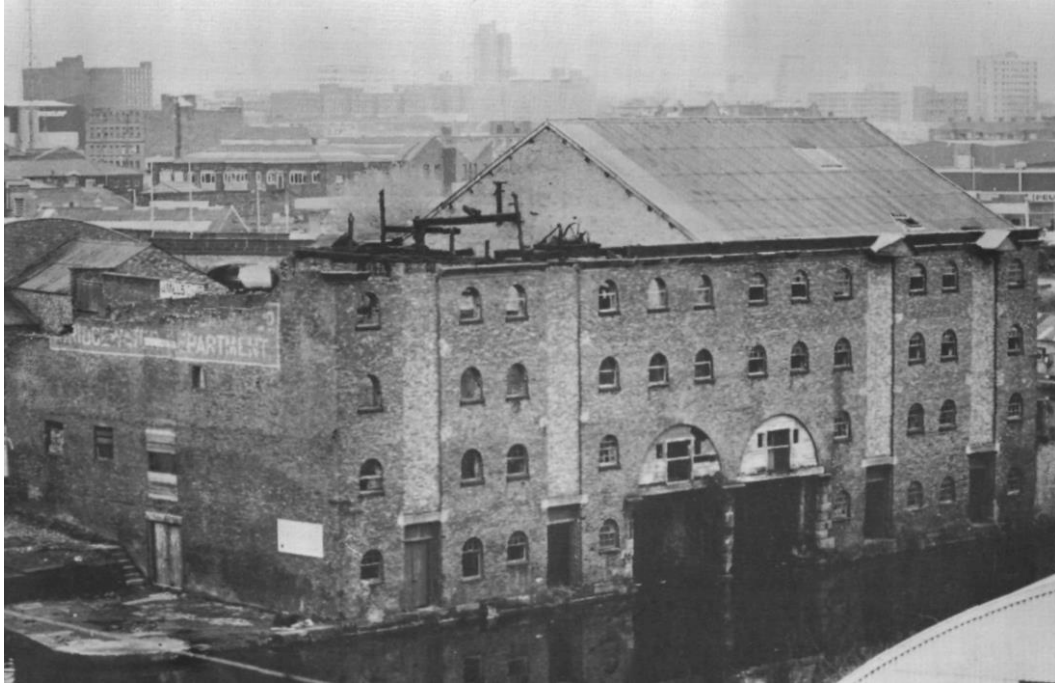
Figure 10: The west (right) and north (left) elevations of the building as seen following the 1971, illustrating the substantial damage to the northern half. Note the relatively unscathed southern half. (Source: http://www.gmau.manchester.ac.uk/pdfs/gmac11.pdf )
