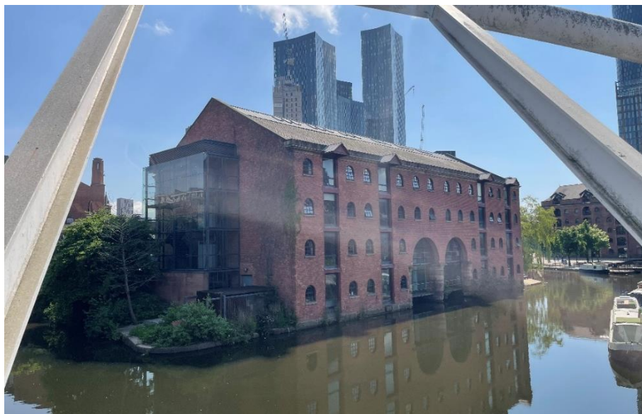
Figure 1: Looking south-east across the Bridgewater Canal towards the western elevation of Merchants Warehouse. (Source: SLHA May 2025)
