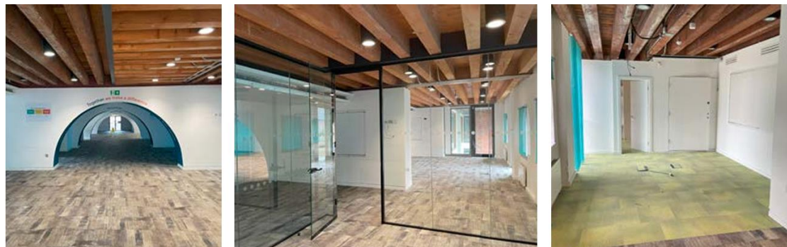
Figure 16: Level 2 as existing, illustrating the addition of modern stud and glazed partitions/flooring etc.
