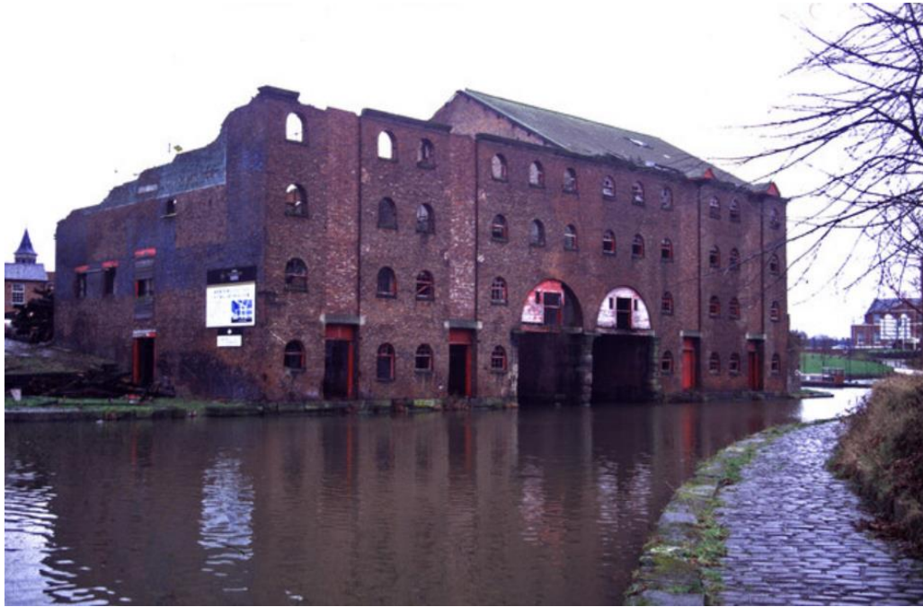
Figure 14: View of the west and north elevations of the Site in 1995 just prior to the building being fully restored as offices. This image clearly shows the deteriorated condition of the warehouse at this time, especially the substantial fire damage to the northern end (left) following the 1971 fire. (Source: www.geograph.org.uk ).
