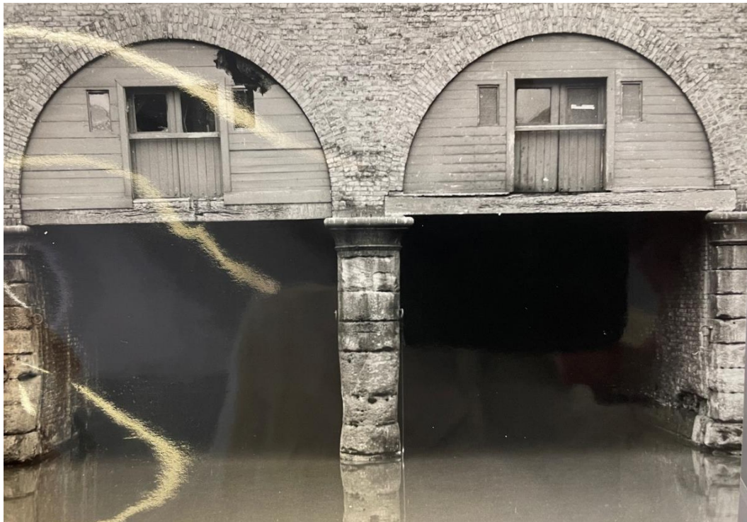
Figure 11: Shipping holes to the west elevation, c.1970s, showing the original open nature of the two openings. (Source: Manchester Central Archives).
