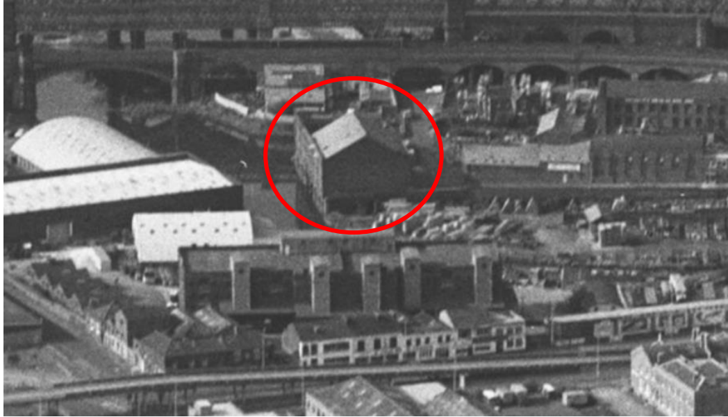
Figure 12: Aerial view of Merchants Warehouse and its local context within the Castlefield Basin, 1979, showing the northern end of the warehouse being roofless and ruinous following the 1971 fire (Source: Britain From Above).
