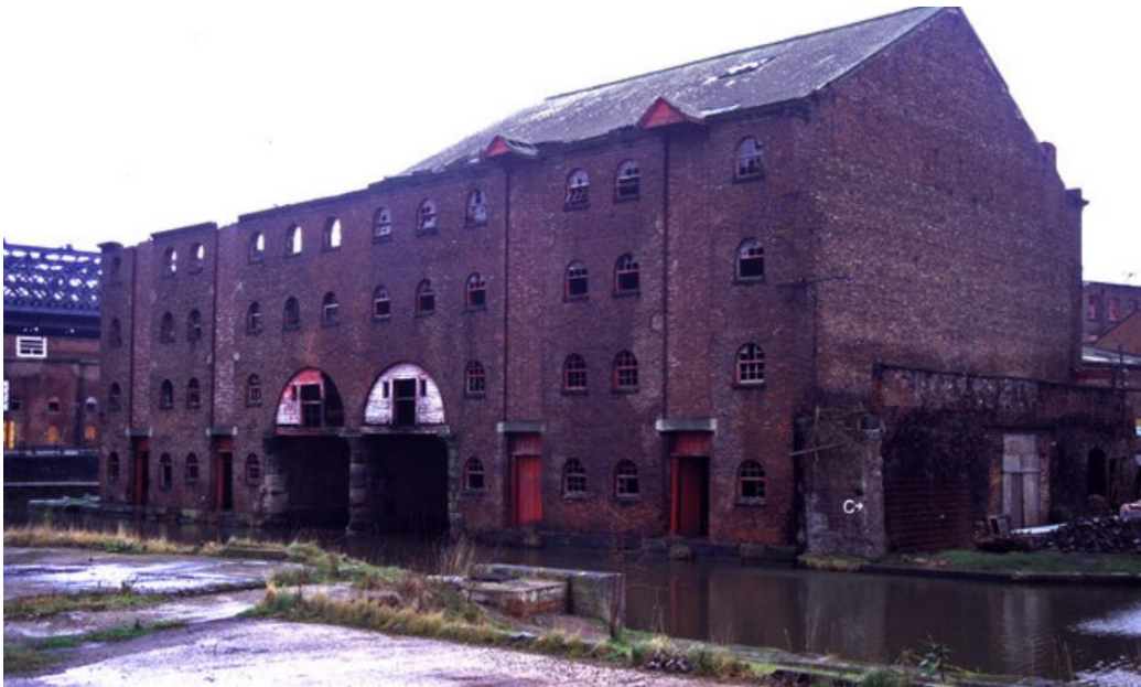
Figure 13: View of the west and south elevations of the warehouse, illustrating their deteriorated condition in 1995 (Source: www.geograph.org.uk ).
