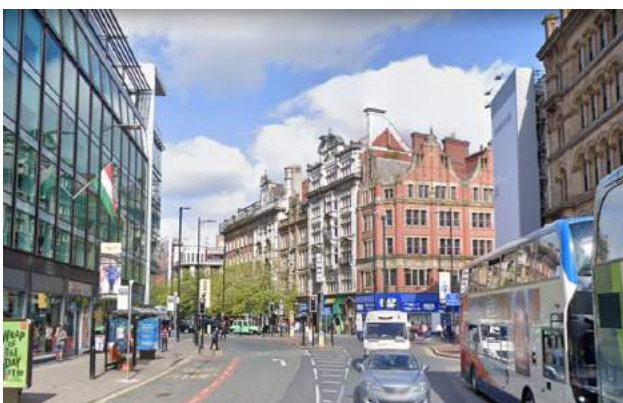
Photograph From Piccadilly Street- South-East of the Building
