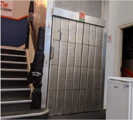
Photograph of Stairwell Lift
