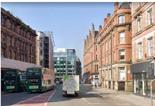
Photograph From Newton Street- North-East of the Building
