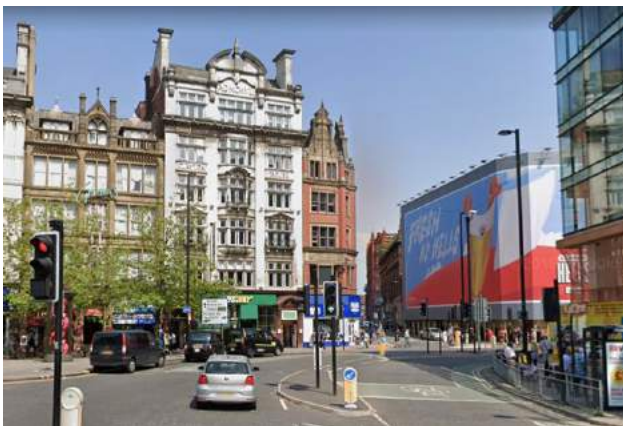
Photograph From Portland Street- South-West of the Building
