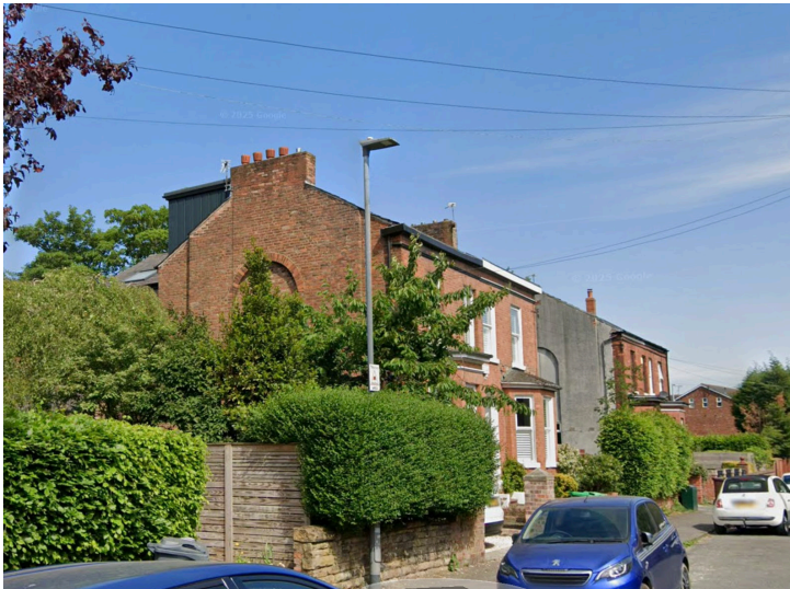
Metal-clad dormer on 46 Whitelow Road (Application 137552/FH/2023) with rendered gable invisible in the background.
