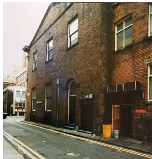
1986 photograph showing the central ground floor window that was subsequently converted into a fire escape for the Pub. The smaller escape door on the righthand side is already in place.
