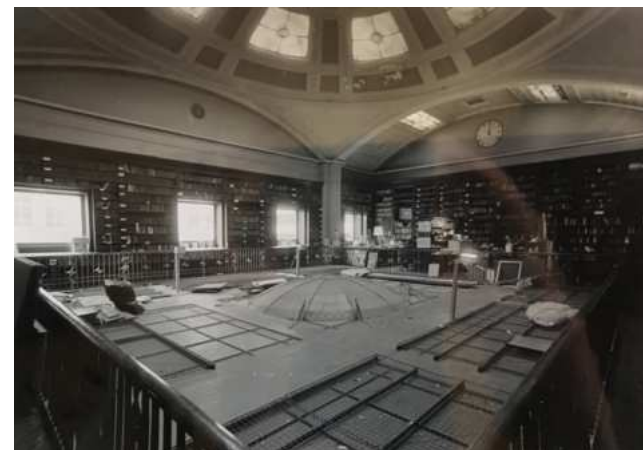
Interior during the 1980s prior to the removal of the glazed ceiling
