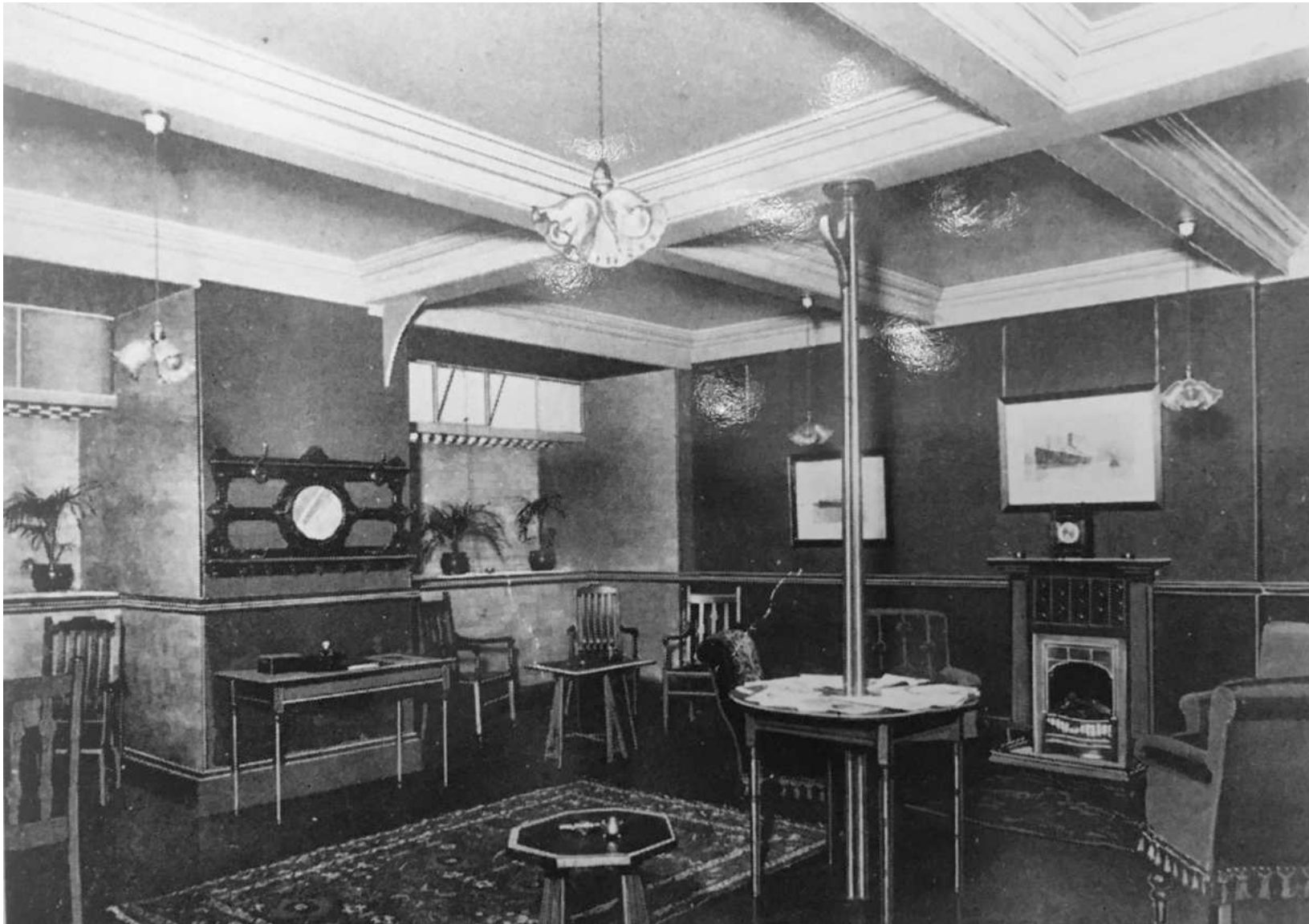
Smoking Room in the Basement, prior to the 1920s conversion
