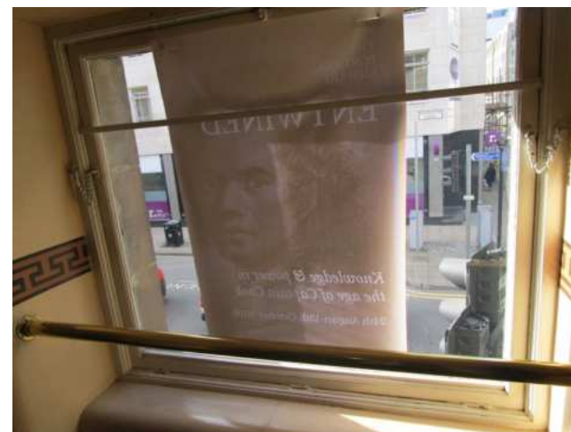
Early 20 th century 1 st floor window onto Charlotte Street
