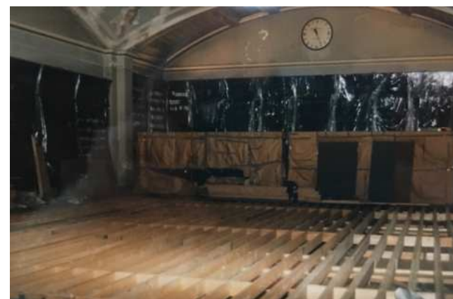
Interior during the 1980s during the work to install a new floor
