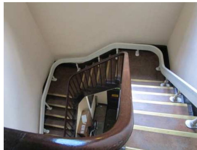
Stair lift in rear stair
