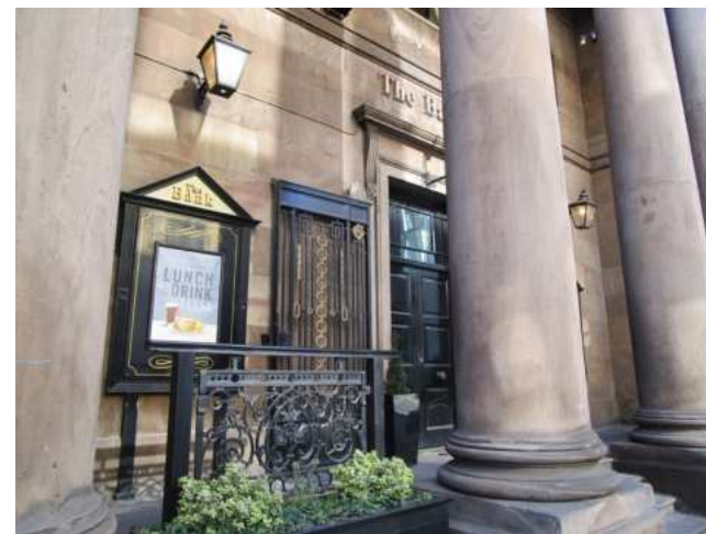
Evidence of the old window openings can be seen at ground floor level
