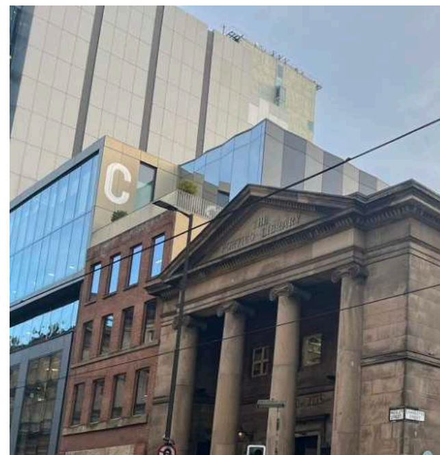
The impact of recent works to the adjacent building
