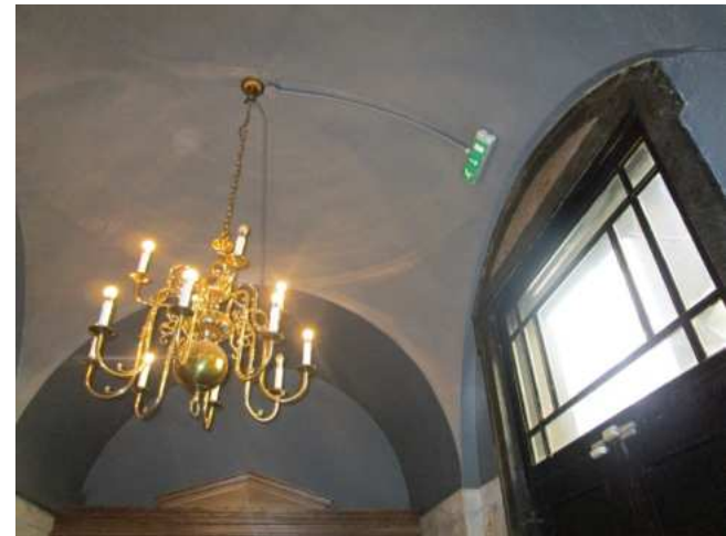
Ground floor entrance vestibule
