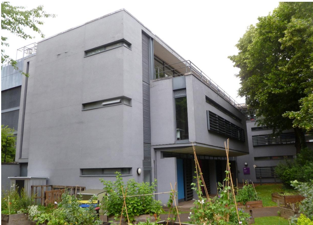
Figure 2.3: Prospect House viewed from adjacent landscaped area.
