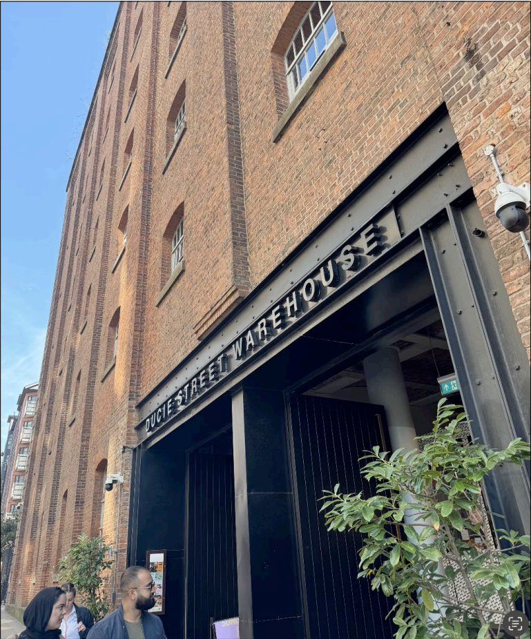
EXISTING SIGNAGE | NORTH ELEVATION
