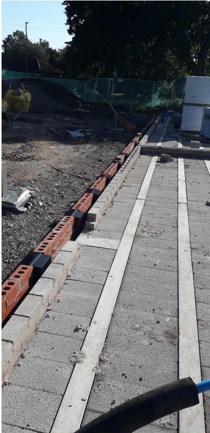
Photograph 2 Swan neck vent being installed into Plots 2 & 3.
