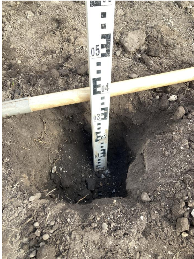
Photograph 8 400mm of topsoil emplaced over granular break layer in VP02.
