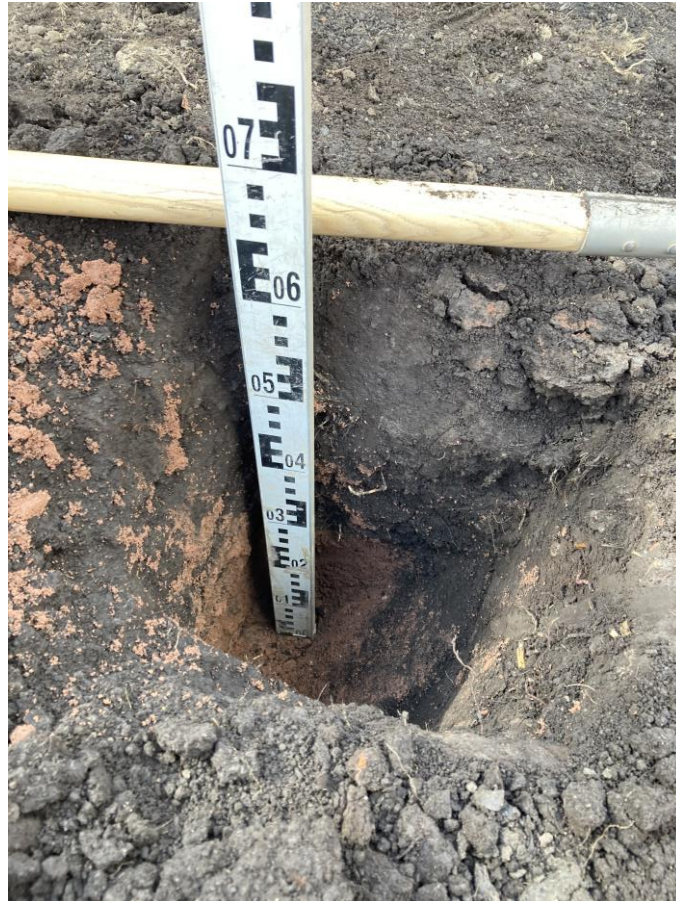
Photograph 12 300mm of topsoil and 350mm of subsoil emplaced in VP04.
