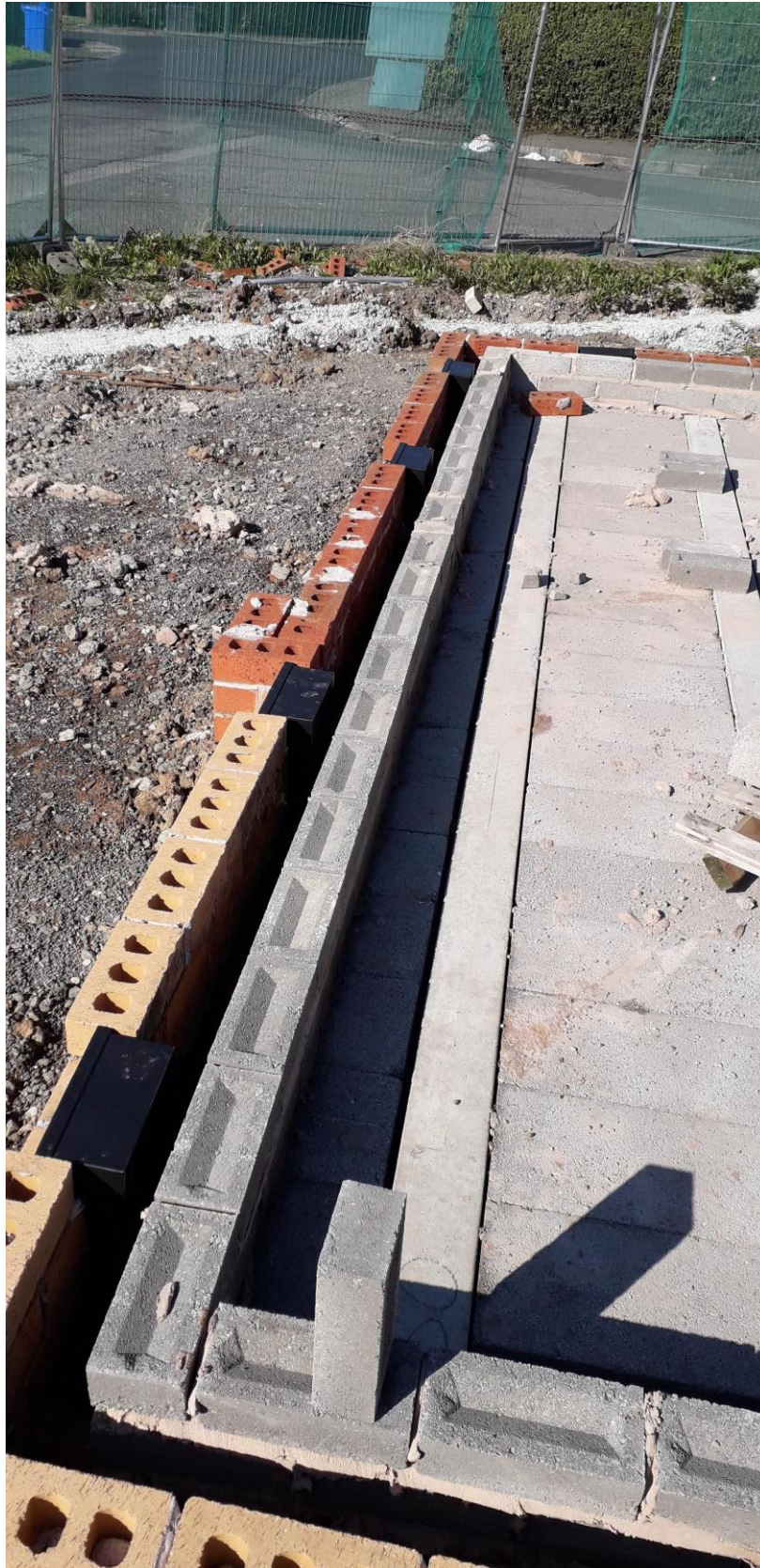
Photograph 1 Swan neck vent being installed into Plot 1.
