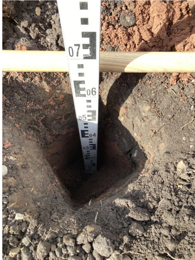
Photograph 6 200mm of topsoil and 450mm of subsoil emplaced in VP01.
