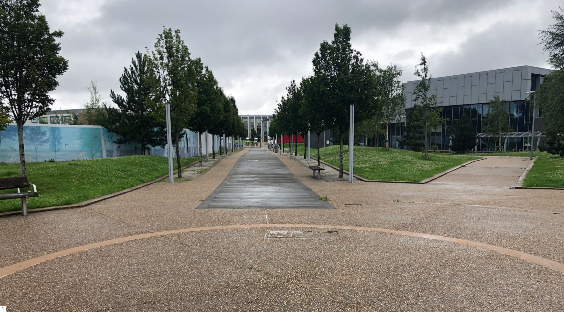
Campus Landscaping - Grey Mare Lane
