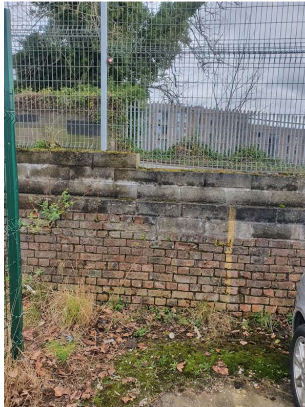
Figure 13 Bridge Abutment Masonry Wall
