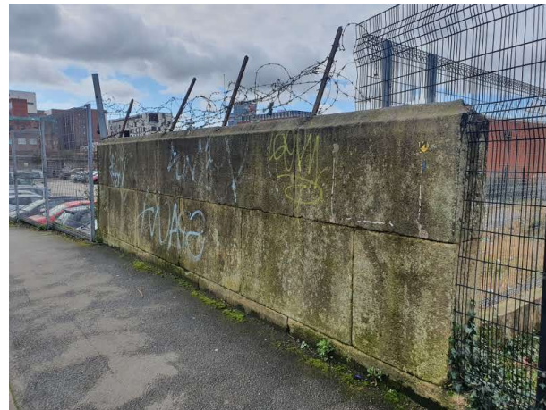
Figure 7. - North Side Bridge Parapet
