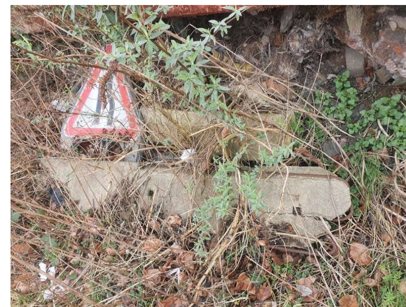
Figure 11 - Stone Encasement Previously Concealing Primary Beam
