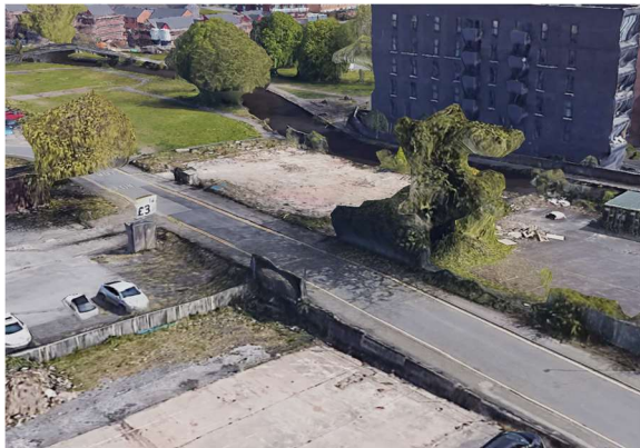
Bridge Ariel View Facing West
