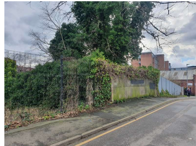
Figure.8 - South Side Bridge Parapet
