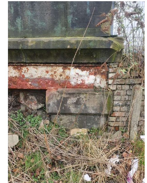
Figure 10. - Bridge Bearing Position
