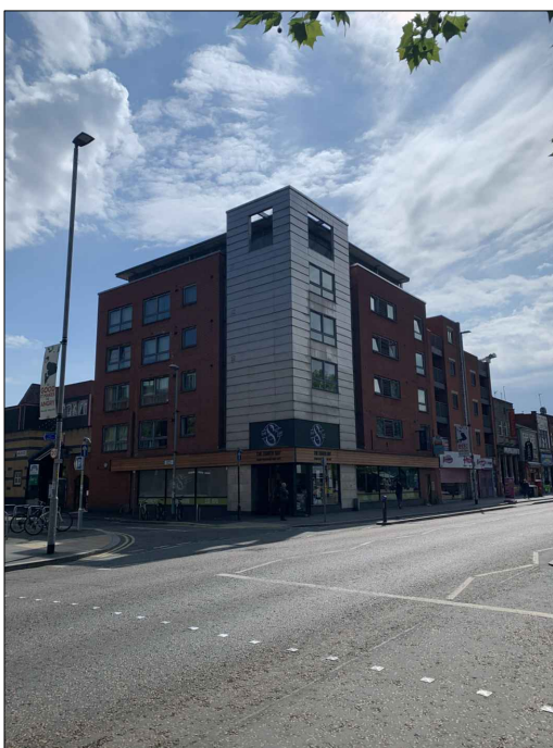
EXITING SITE IMAGE (1)
