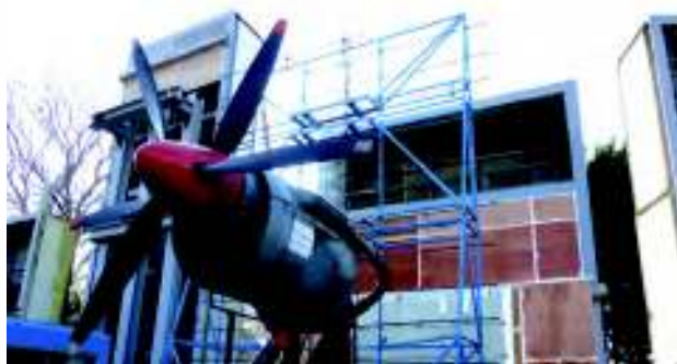
Dynamic water tightness testing at Vinci Technology Centre
