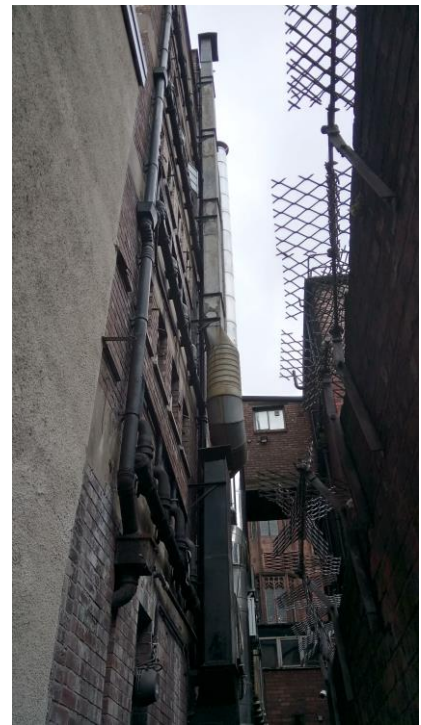
Figure 5: Flues to rear of premises on Deansgate
