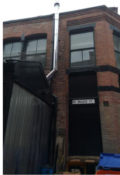
Figure 3: Flue on Back Bridge St
