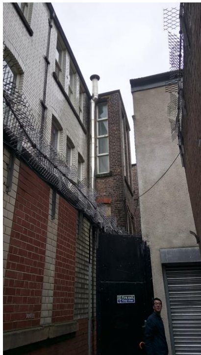
Figure 4: Flue to rear of property on Bridge St
