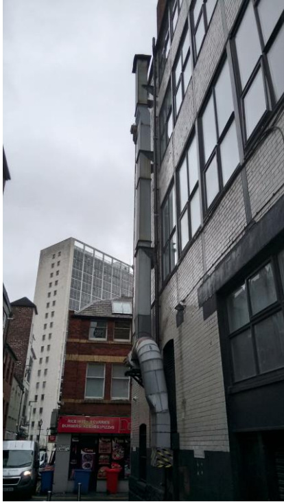
Figure 2: Flue on Back Bridge St
