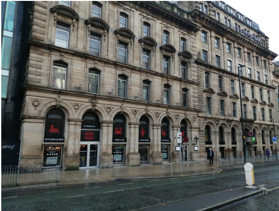
Figure 5.5: Jamboree signage at ground floor level of the Portland Thistle Hotel.
