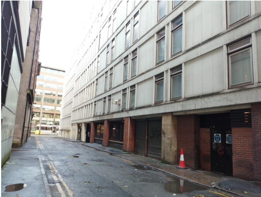
Figure 5.8: Rear elevation of the Portland Thistle Hotel.
