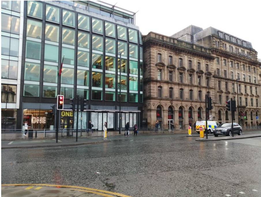
Figure 5.4: The site read in conjunction with the front elevation of the Portland Hotel.
