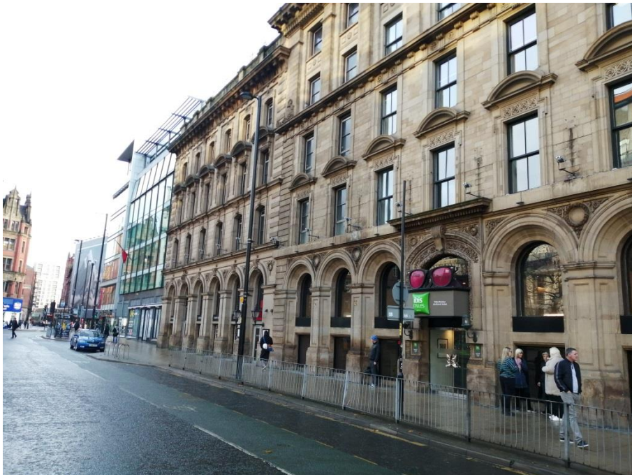
Figure 5.6: Ibis Hotel signage above the front entrance of the Portland Thistle Hotel.
