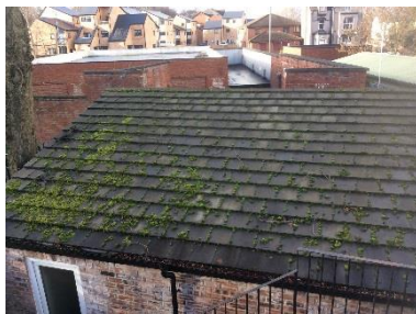
B3; sloping tiled roof
