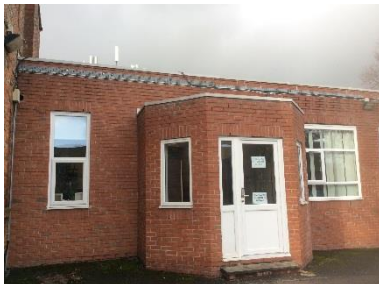
B1; flat roofed building
