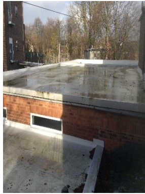
B1; bitumen roof
