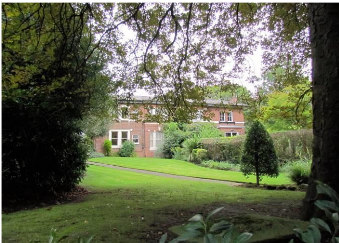
Mid-19 th century Semi-detached Houses
