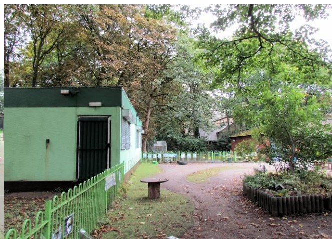
Late 20 th Century Building
