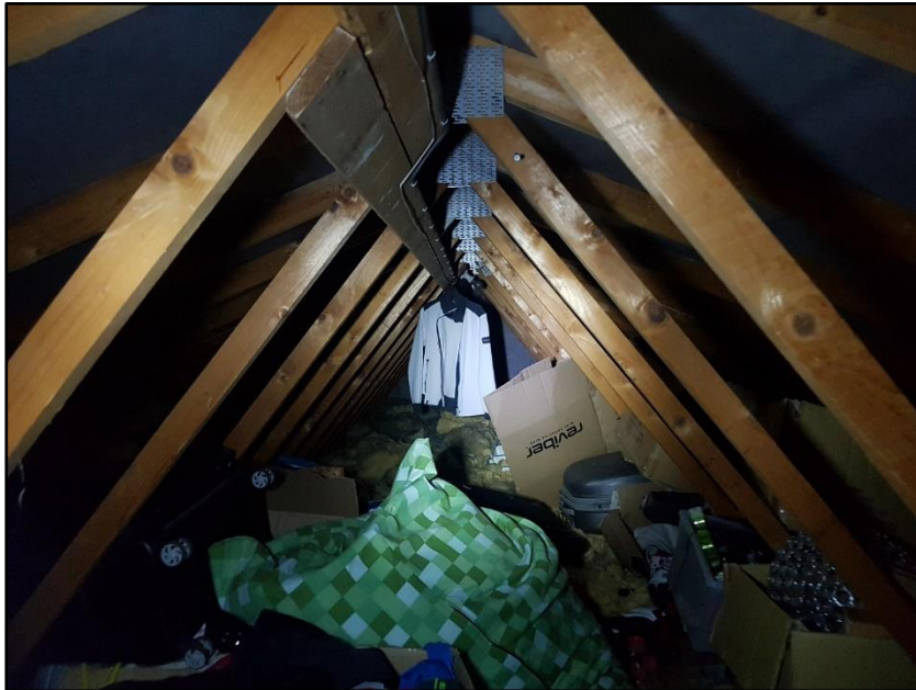
Photograph 6 showing the roof void
