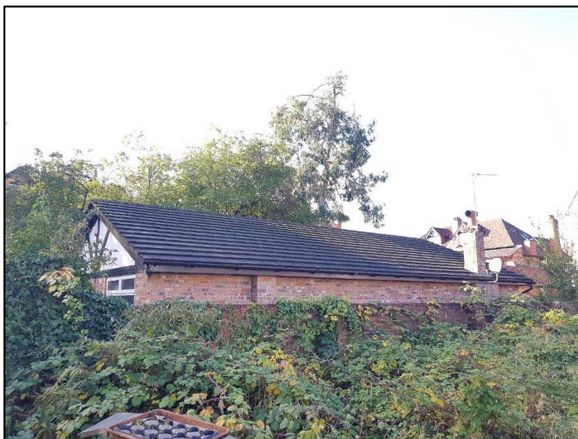
Photograph 5 showing the roof of the building
