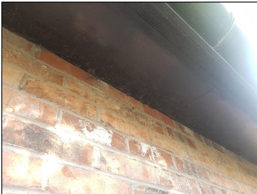
Photograph 4 showing the wooden soffit boards
