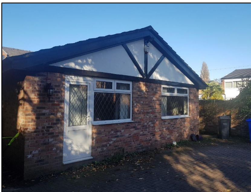
Photograph 1 showing the eastern gable end
