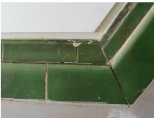
Image showing an existing shadow gap detail within the building, the principle of which is to be followed for any new partitions.
