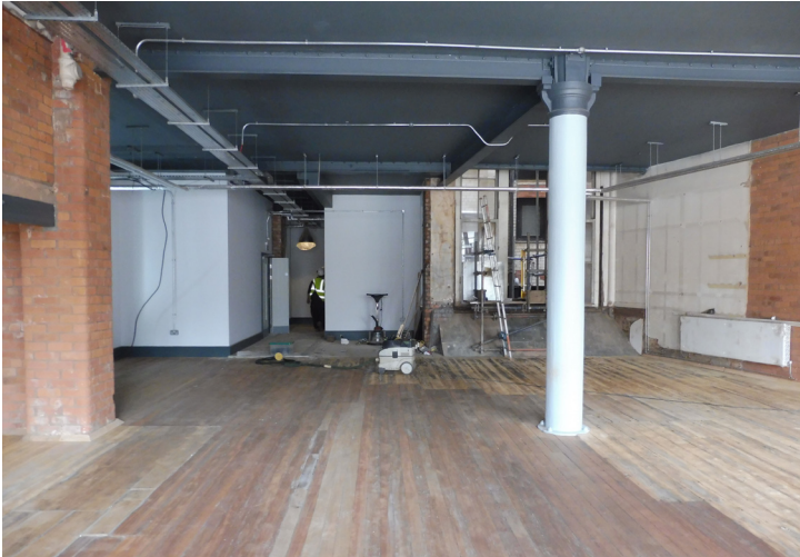
Image showing the existing ground floor with exposed timber floor, columns, brick walls and ceiling, following the strip-out works completed as part of a previous application (Ref. 115335/LO/2017).
