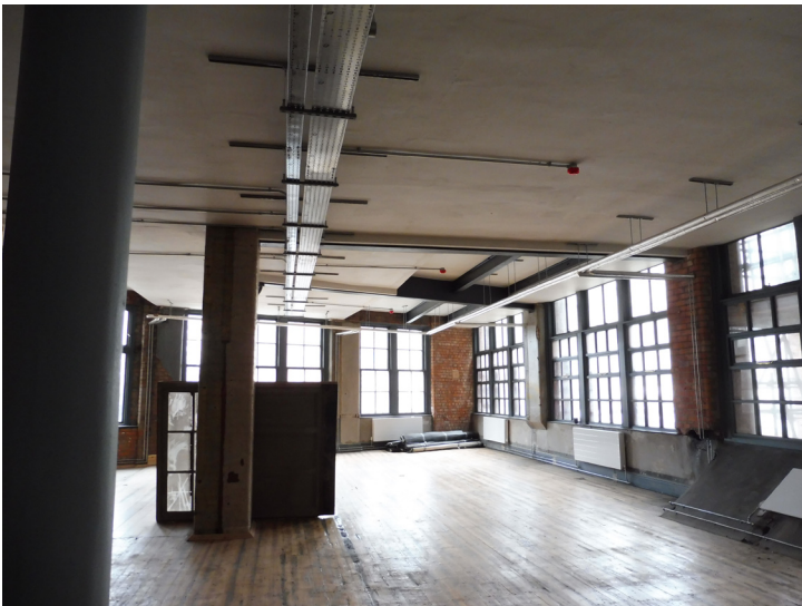
Image showing the existing first floor and ceiling following the works completed as part of a previous application (Ref. 115335/LO/2017).
