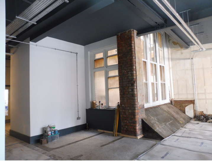
Image showing the existing partitions and ground floor area where the new kitchen is proposed to sit.
