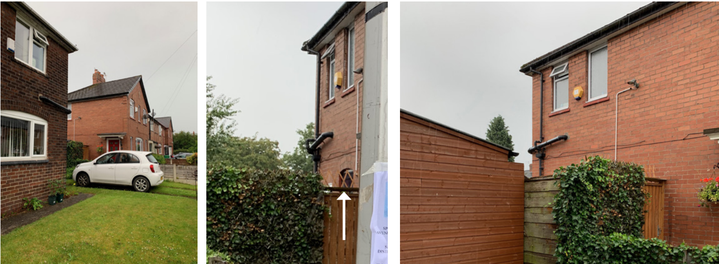
Photos of 21 Burrows Avenue showing the existing openings on the side elevation facing the application site
