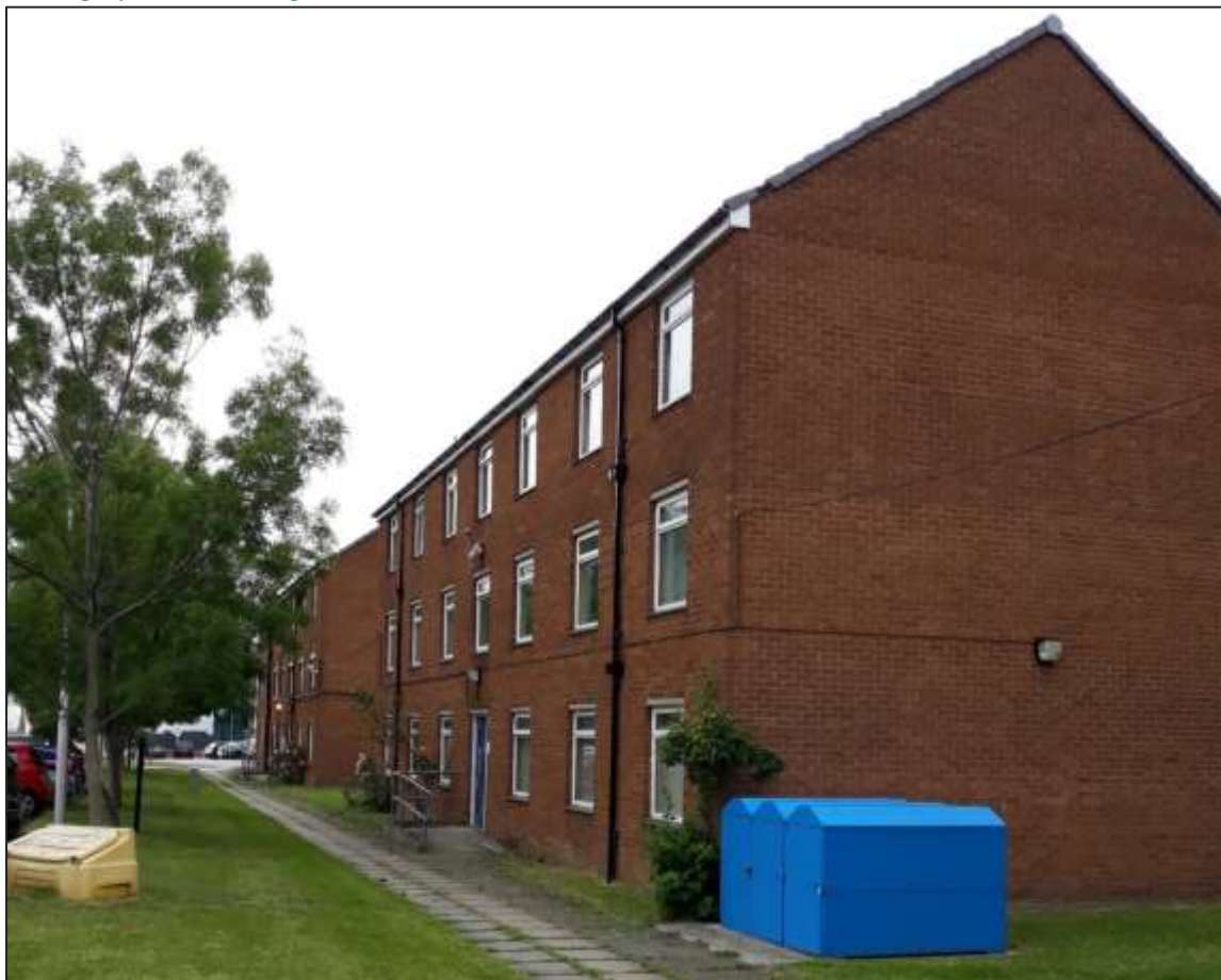
Photograph P1: Building B01
