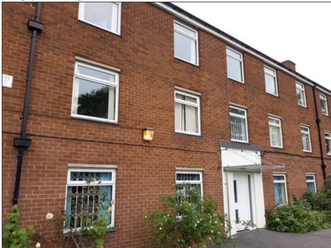
Photograph P2: Building B02
