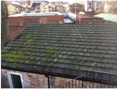
B3; sloping tiled roof
