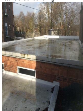
B1; bitumen roof
