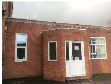
B1; flat roofed building
