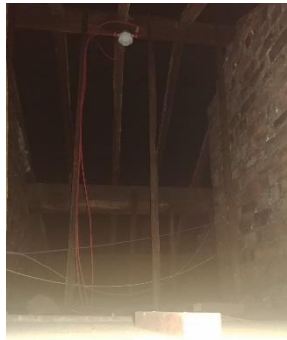
B2; Loft void above corridor
