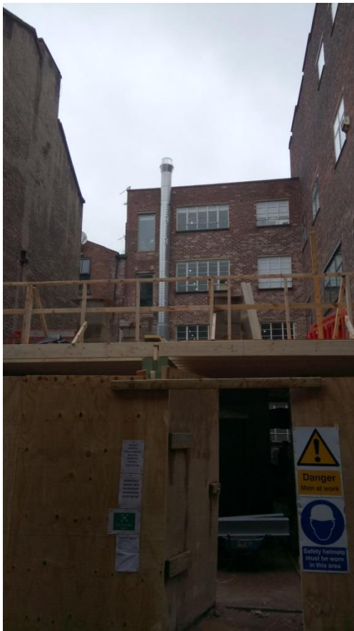
Figure 4.1: View of the extraction system from Wood Street looking across the gap site (June 19). Works have since continued and the flue is no longer visible.
