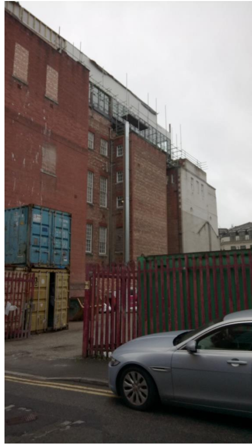
Figure 4.3: View of similar extraction system nearby on the car park west of the site between Wood Street and Bridge Street.
