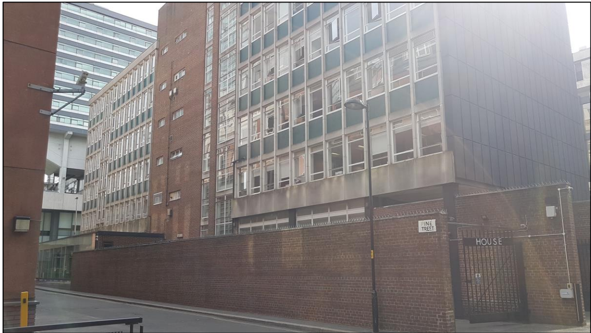
Figure 4: View of Pine Street elevation and New York Street elevation (blank gable) of Faulkner House.
