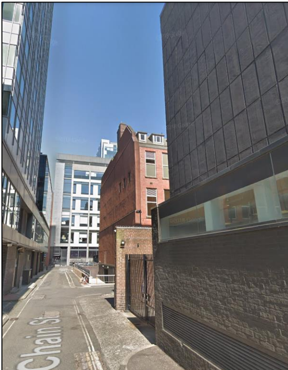
Figure 9: View showing Faulkner House in the context of 'Telephone Buildings' looking along Chain Street.
