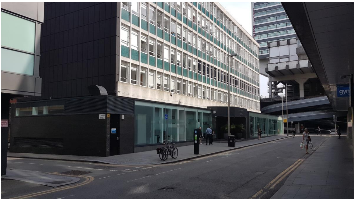
Figure 3: View of the Faulkner Street elevation and the existing entrance area.
