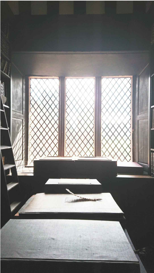
⑮ Window soffit paneling has been over-boarded with 2-3 mm hardboard but frame remains intact.
