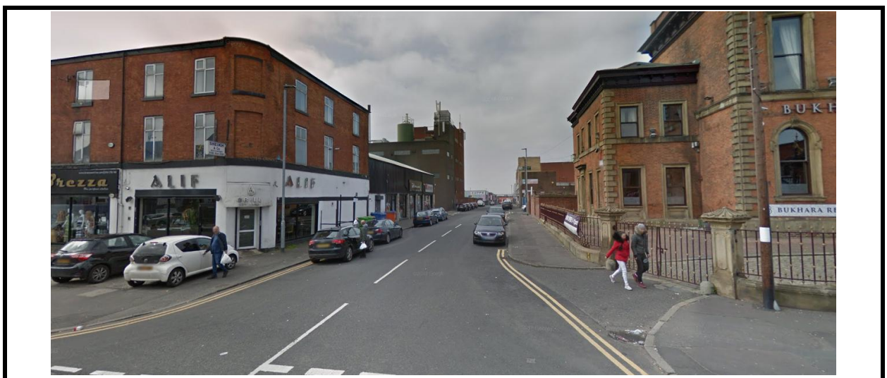
View along Knowsley Street showing on street parking
