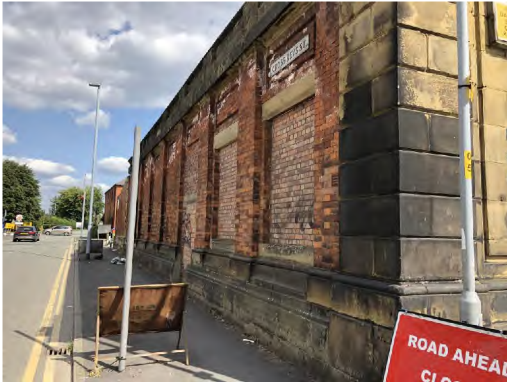
Figure 6 – View of existing boundary from Cross Keys Street/Goulden Street Junction
