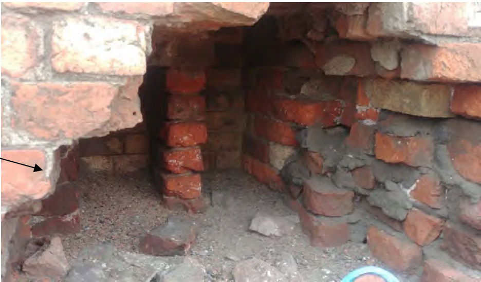
Approximate wall thickness 950mm
