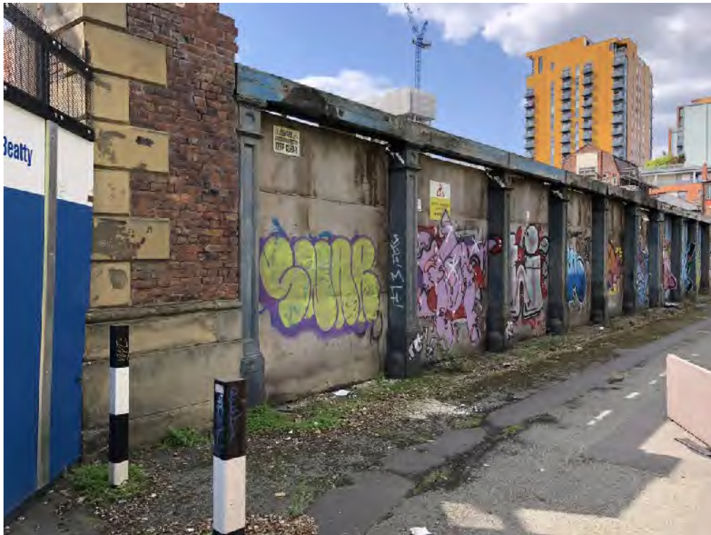
Figure 2 – View of existing boundary from the North Elevation Alleyway.
