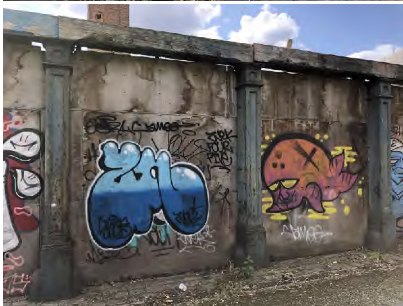
Figure 3 – Cast Iron Columns to be kept, repaired and built into new scheme
