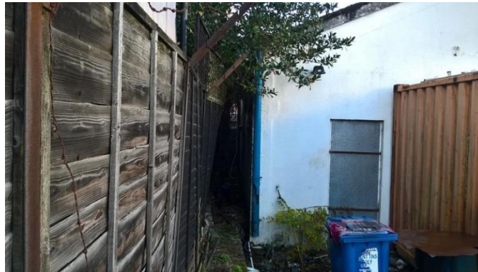
Plate 38: Southern Side of Building 2.
