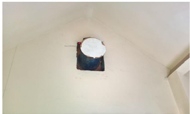
Plate 25: Old Blocked-off Fan Unit in the Southern Elevation of the Laundrette Office.
