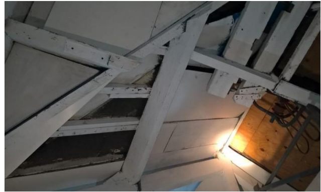
Plate 34: The Wooden Boards which were Intact but Lifting.
