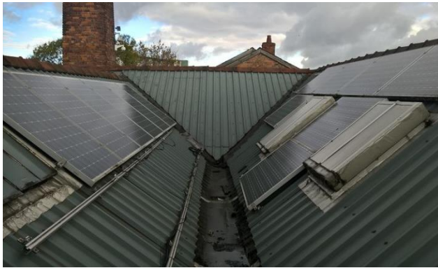
Plate 12: The Roof Walkway with Corrugated Metal Sheeting, Skylights and Solar Panels Present.
