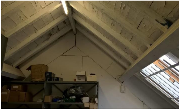
Plate 33: The Wooden Boarded Ceiling of the First Floor.
