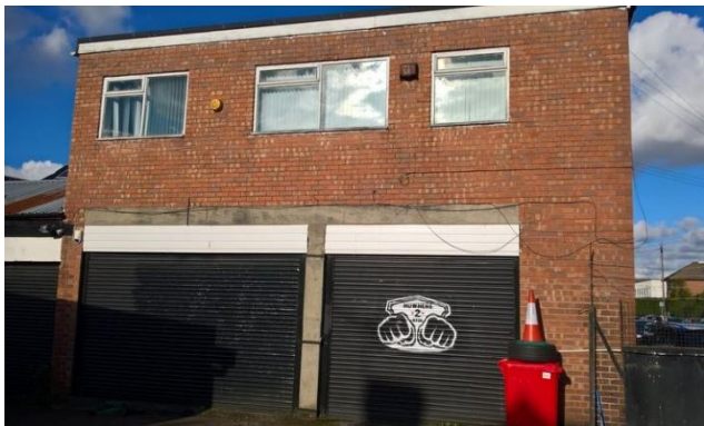
Plate 1: Flat Roofed, Two-Storey Section to the South-east.
