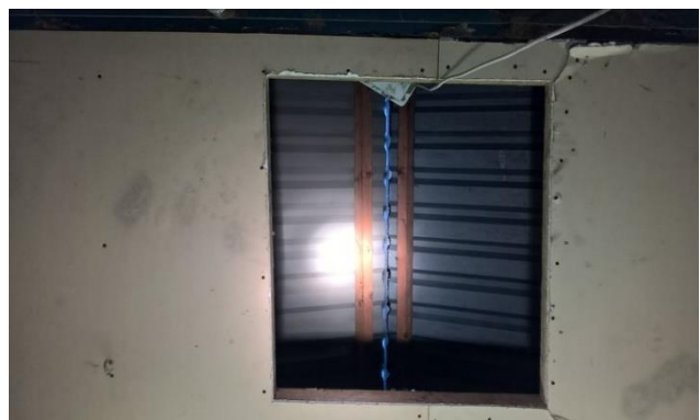
Plate 27: Metal Corrugated Roof Seen Through the Loft Hatch.
