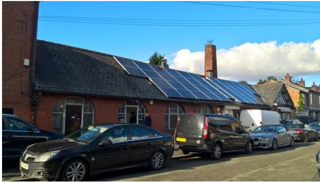
Plate 6: Eastern Elevation of Building with Solar Panels.
