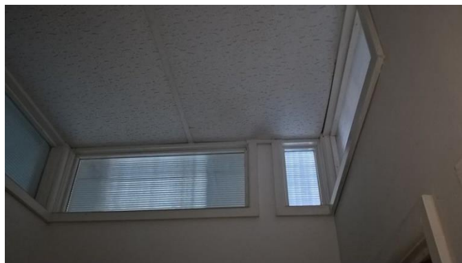
Plate 19: The Roof in the Hallway Outside the South-eastern Offices.
