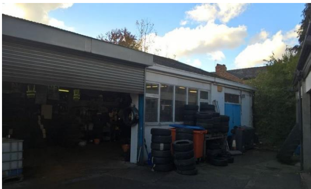
Plate 39: Northern Aspect of the Workshop with the Metal Shutter Door and Intact Windows.
