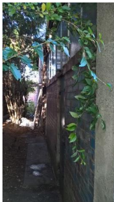
Plate 4: Scrub Vegetation on Western Side of the Building.
