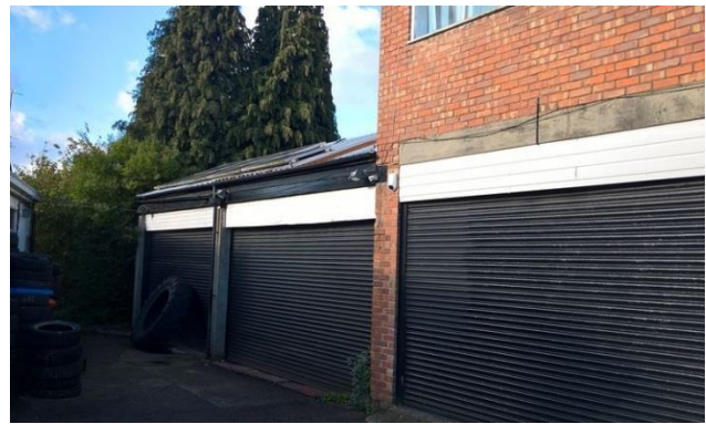
Plate 2: Corrugated Pitched Roof Section to the South-west with Metal Shutter Doors.
