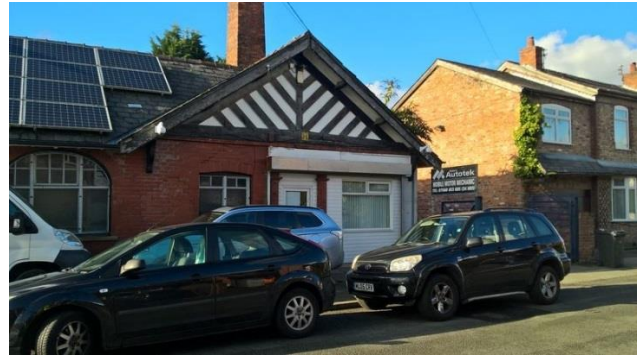
Plate 7: North-eastern Section of Building with Mock-Tudor Gable and uPVC Cladding.
