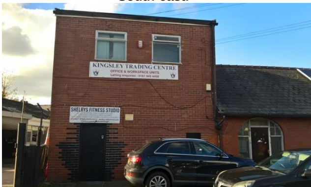
Plate 3: Eastern Elevation of the South-eastern Section.
