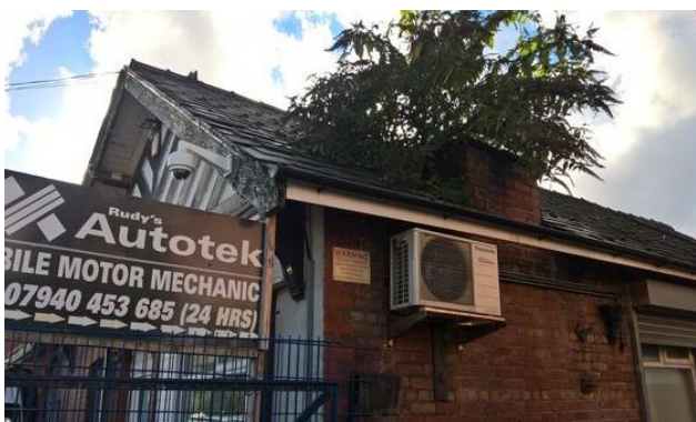
Plate 9: The Northern Pitched Roof Section.
