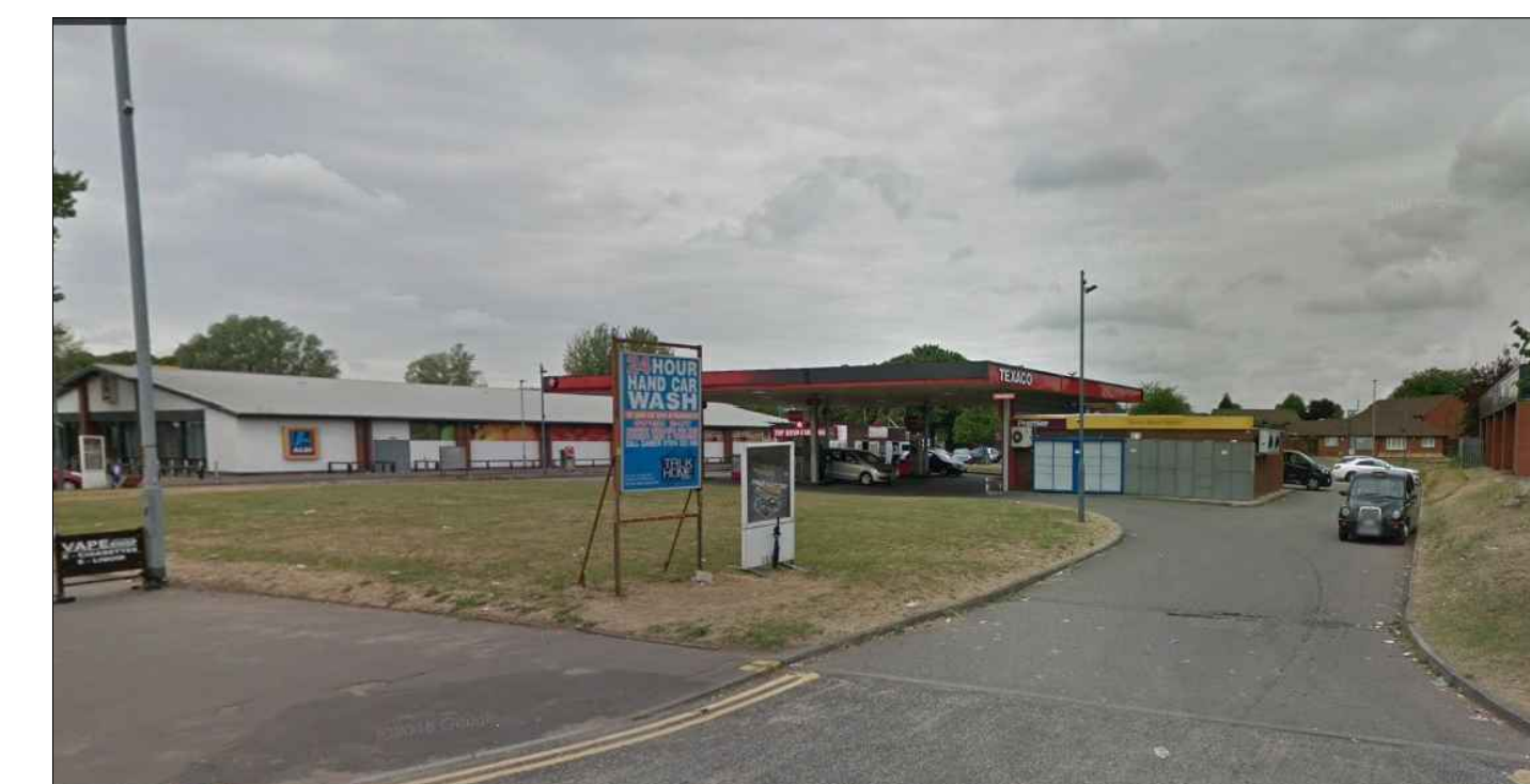
SITE PHOTO VIEW 2
