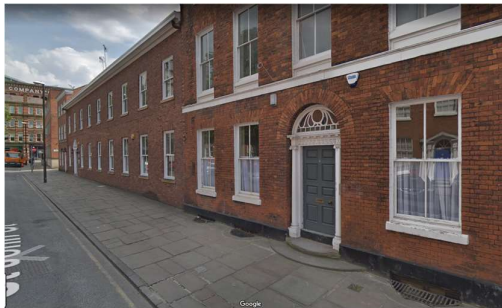
View of 13 St John street facing east (towards Deansgate)
