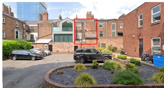
View of 13 St John Street from the rear (bordered in red)
