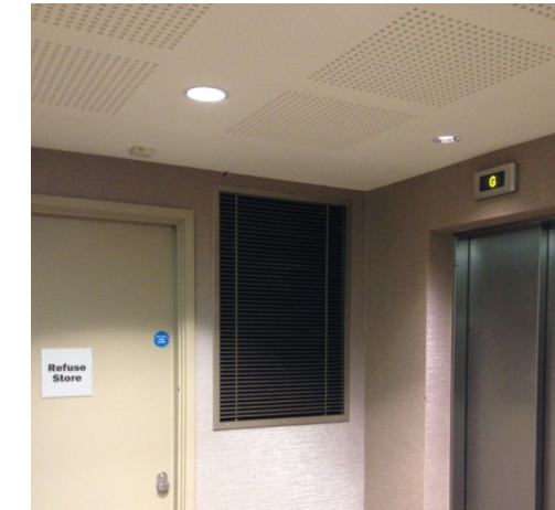
Typical smoke ventilation grille
